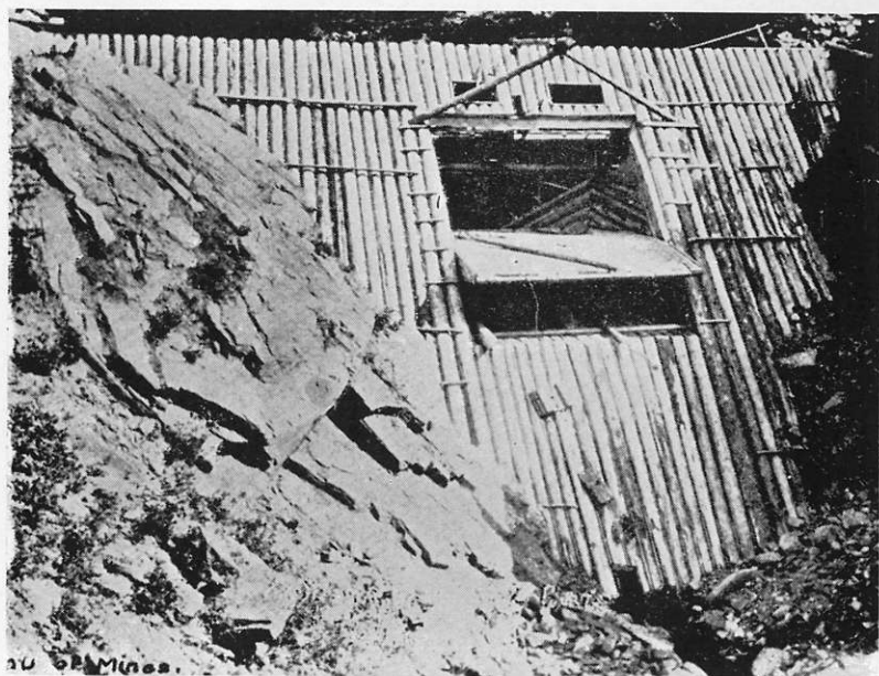
Weaver Creek—A Boomer-gate for Placer-mining.
