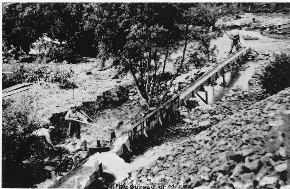
Spruce Creek, Atlin—Shovelling in to Sluice.
