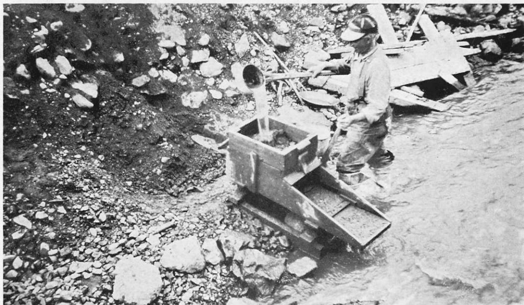
Spruce Creek, Atlin—Method of washing Gravel with Rocker.
