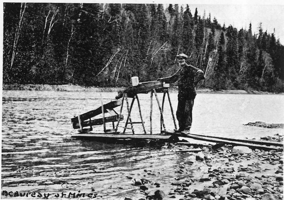
Fraser River—A Long-tom in Use for Sluicing Gravel.
