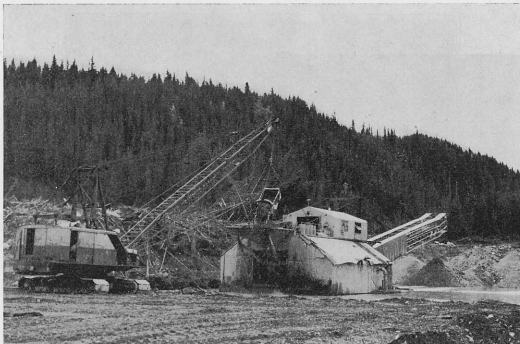
Dragline dredge, consisting of dragline shovel and floating washing plant.
