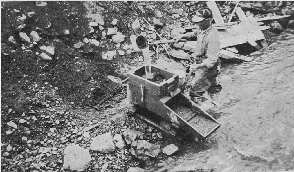
Washing gravel on Spruce Creek with a rocker.
