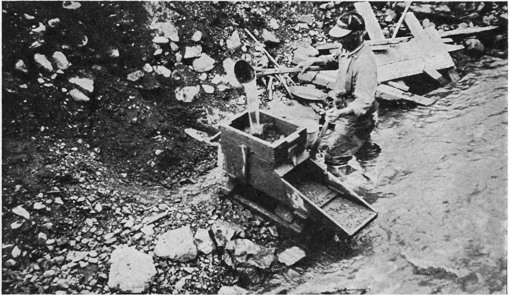
Washing gravel with a rocker, Spruce Creek, Atlin.
