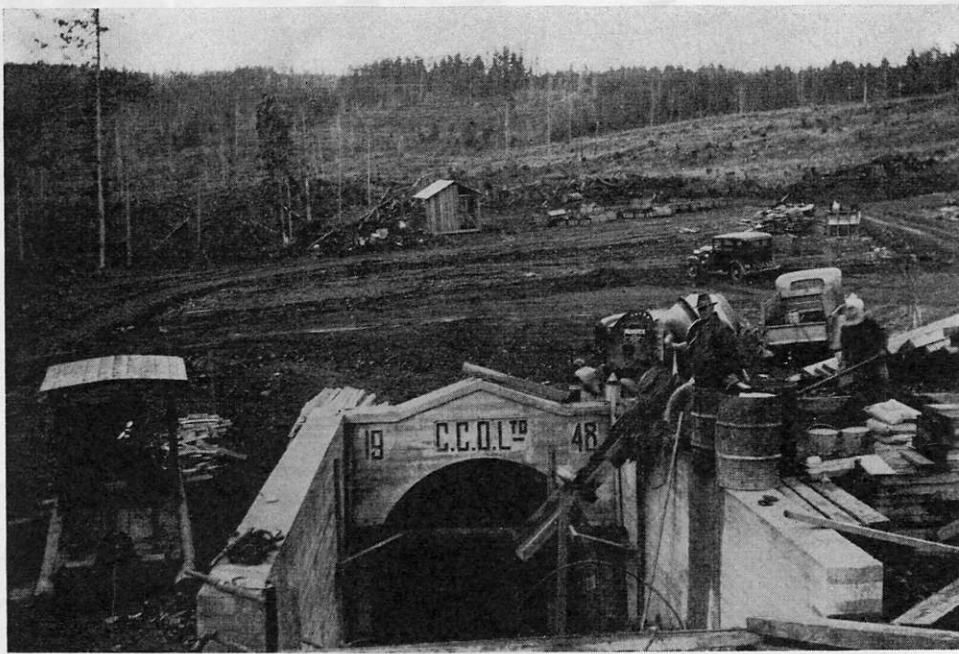
Entrance to main-slope portal, Tsable River coal mine.
