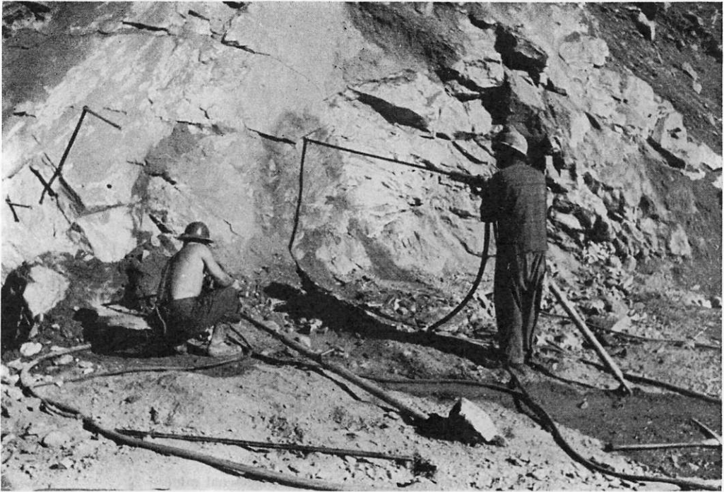
Jack-leg drilling in glory-hole at Reeves MacDonald silver-lead-zinc mine.
