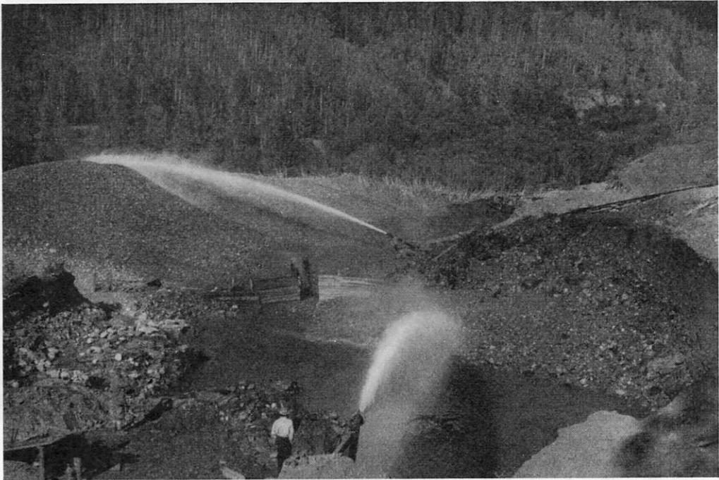
Hydraulic mining on Wright Creek, Atlin.
