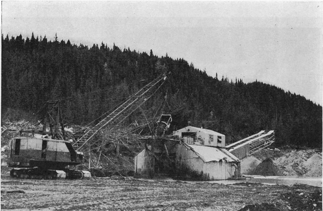
Dragline dredge, consisting of a dragline shovel and floating washing plant, Pine Creek, Cariboo.
