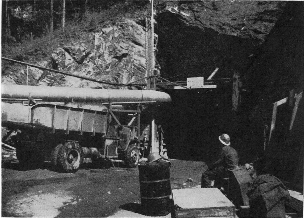
Truck entering portal of Dodger 14- by 15-foot trackless adit.
