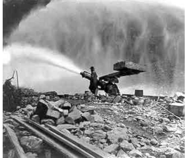
Figure 10. Consolidated Cariboo Hydraulic Mining Company's 15-centimetre (6 inch) monitor in 1896. (British Columbia Archives and Records Service, HP 99924).
