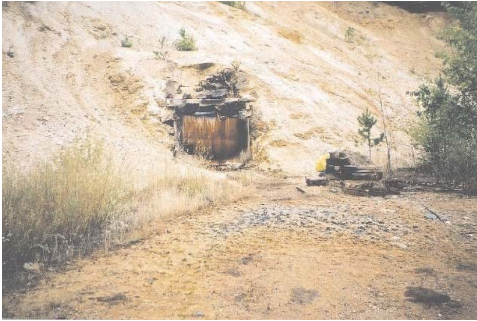
Photo 24. Homestake (Kamad) lower adit. Note white salts in front of the adit.
