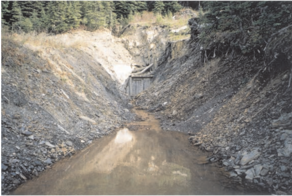
Photo 68. Drainage, heavy in iron precipitate flowing from the Warspite lower adit.
