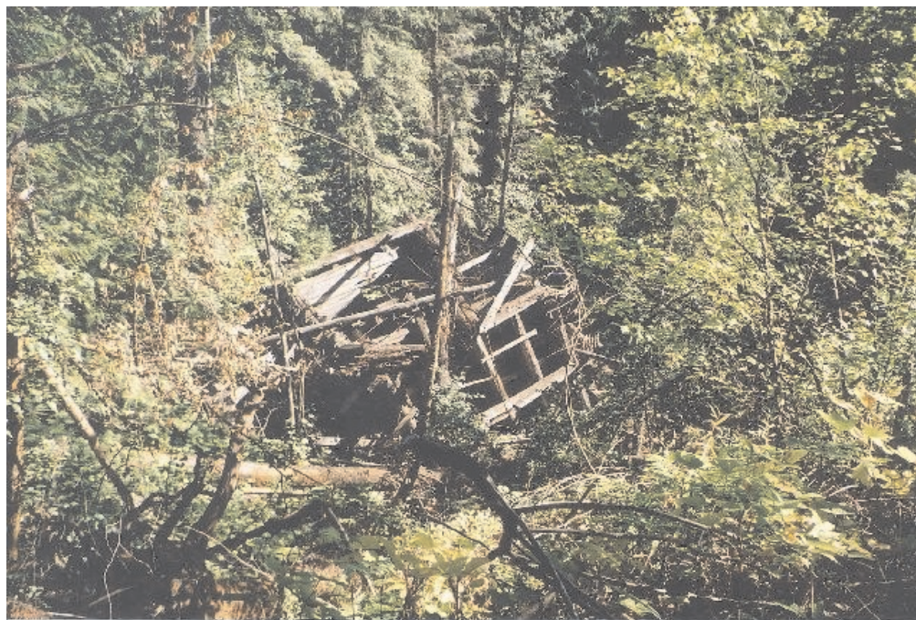
Photo 40. Collapsed tram load out station at Highland mine site.
