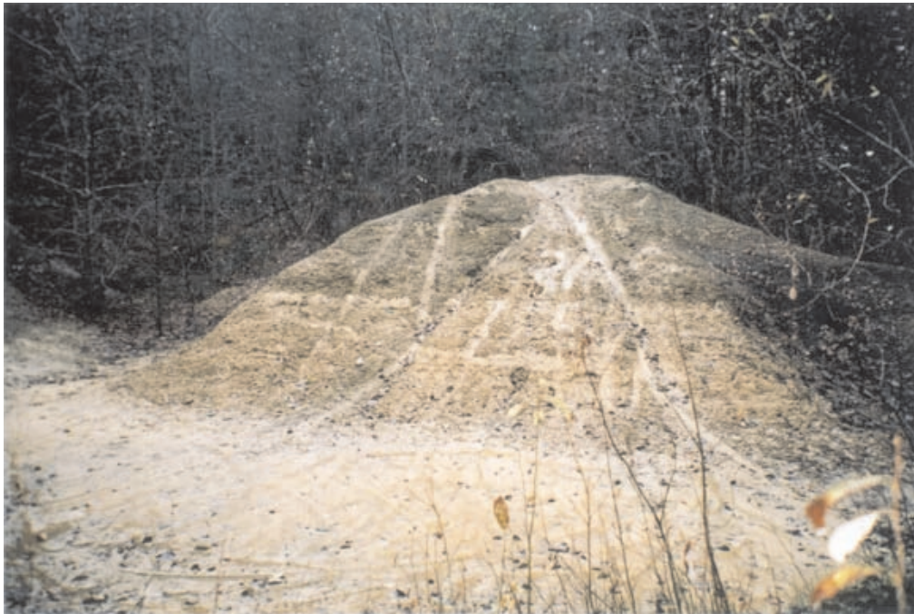
Photo 78. Blue Grouse upper tailings facility.
