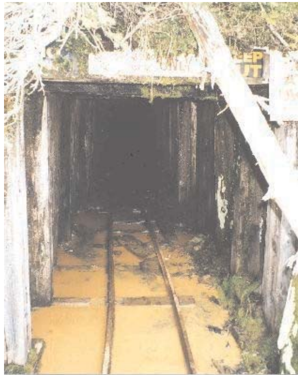
Photo 14. Dunwell 1200' portal. The drainage was sampled.
