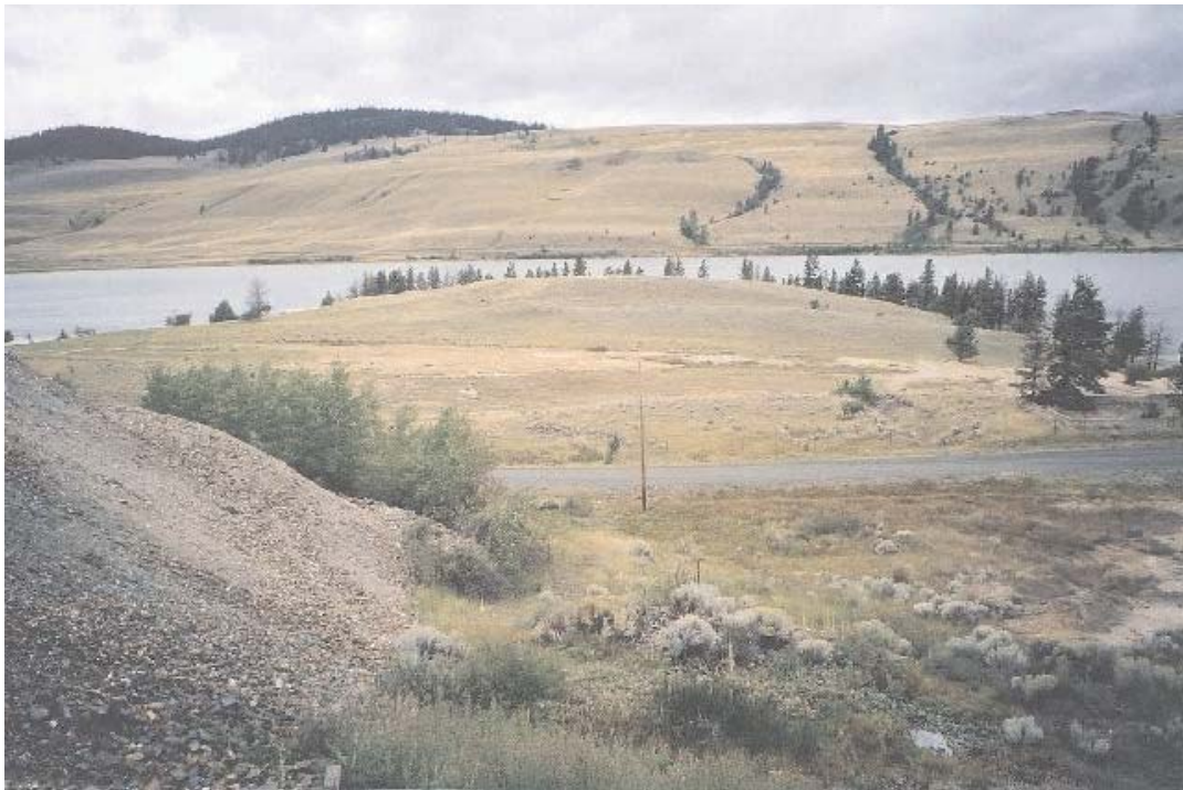
Photo 26. The partially revegetated Enterprise tailings facility (across the road). Dump is in foreground.
