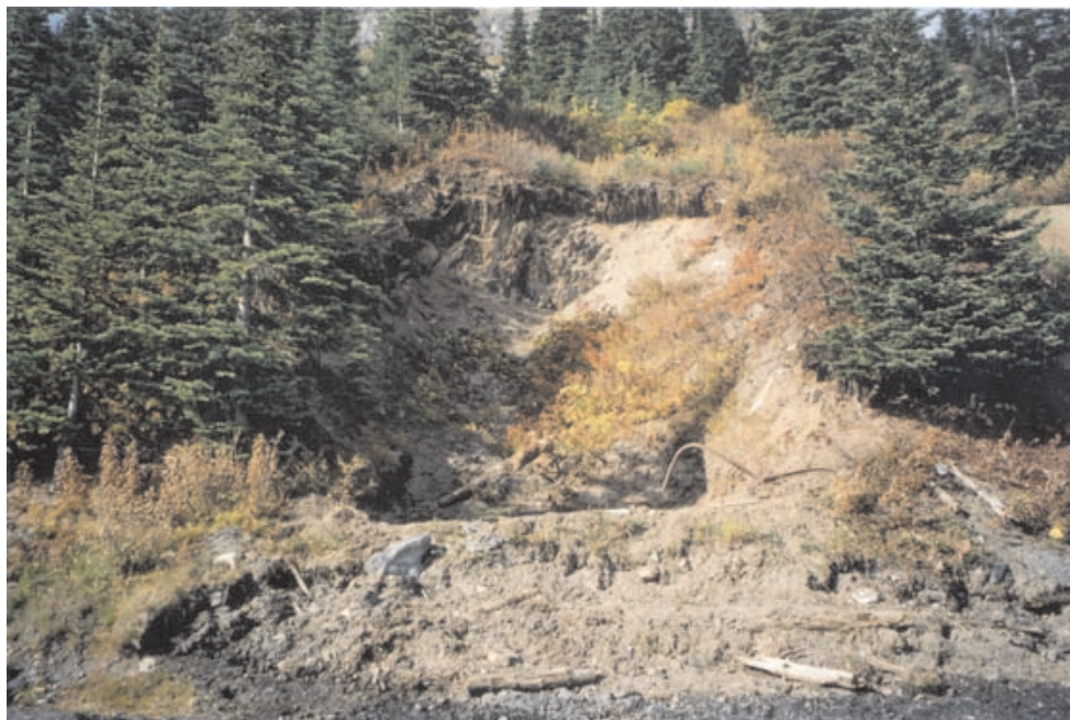
Photo 57. Backfilled portal at Takla Silver mine site.
