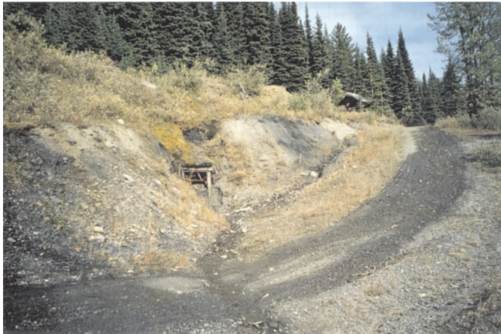
Photo 66. Lower portal at the Jane (Snowshoe) mine site. Note upper adit drainage path at the base of the bank and the hut at the road hairpin.
