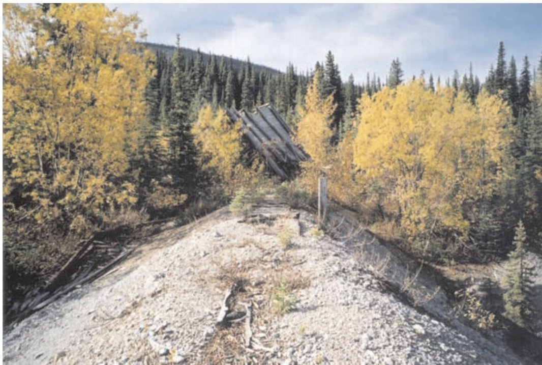
Photo 58. Bralorne-Takla dump and shaft headframe.
