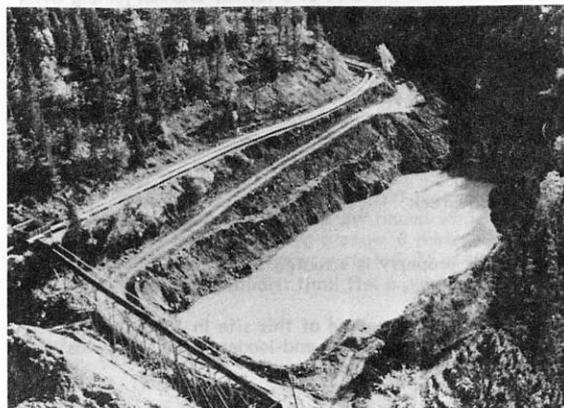
View of narrow, steep-sided Spruce Creek valley at site of Irving operation. The deep cut is visible in the background. In the foreground, the cut is being used as a settling pond.
