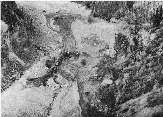
View of the T. Sandor mining operation on Ruby Creek. The steep walls of the valley, and the large size of some of the boulders encountered in the gravel are noticeable.
