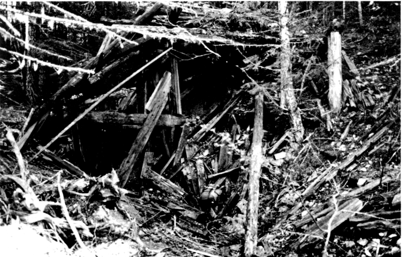
Figure 6-4. Old mine workings. Old mine workings are dangerous to explore. There will almost certainly be records of workings as elaborate as this. Look around nearby dumps to see what may have been mined.
