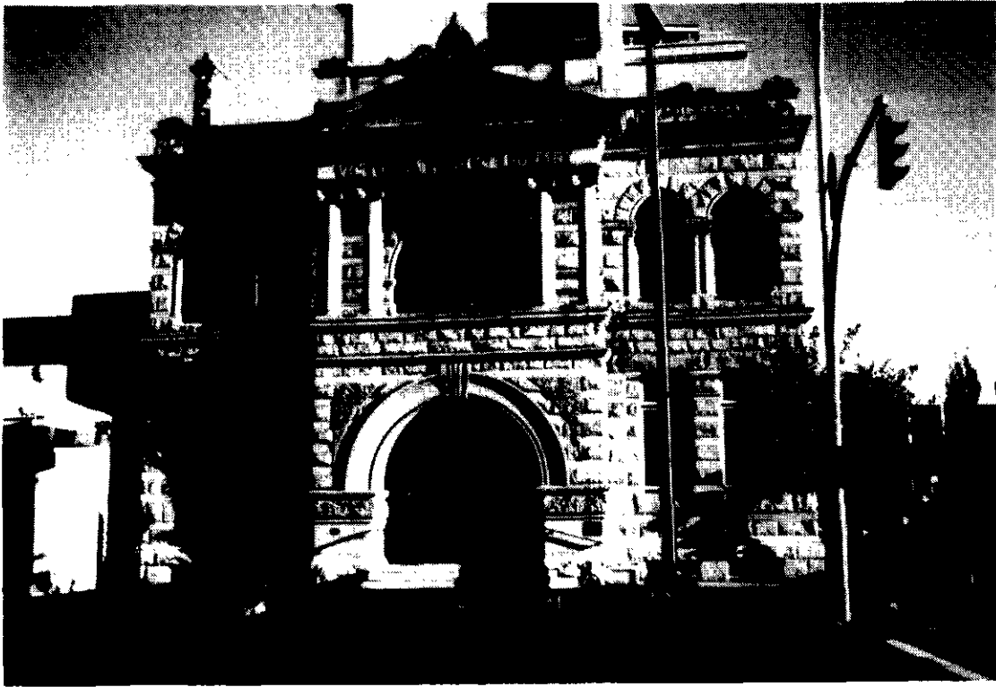
Plate 3-5-1. The old Victoria Public Library (Carnegie Library), designated a heritage building, was constructed using Saturna Island sandstone.
