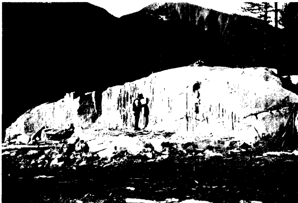
Plate 3-6-1. Working face — Knight Inlet Quarry (92K/12W).
