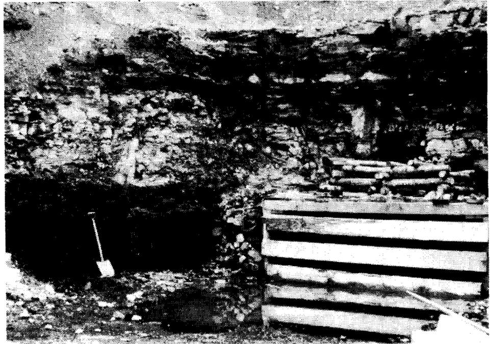
metre pattern. A slope was driven 4.6 metres wide down the full dip of the bed, until unoxidized coal was reached at 18 metres from the portal (Figure 6). At that point a short room was turned off to provide a bulk sample site in 1.34 to 1.37 metres of coal and to test roof conditions across wider spans. There has been no further work on the Chute Creek 'A' bed in regards to testing or to mine planning.
