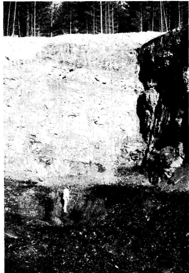
Plate 1. Highwall of the Quinsam colliery, Pit 2N, looking to the north. The person in the photo is standing on the No.1 coal bed.
