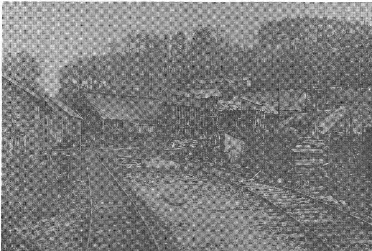
Plate 26. View of upper terminus of the Lenora, Mt. Sicker Railway on Mount Sicker. The ore bins, dump and buildings of the Lenora mine can be seen in the background. The Tye mine appears up the hill to the right (Provincial Archives photograph HP58002).
