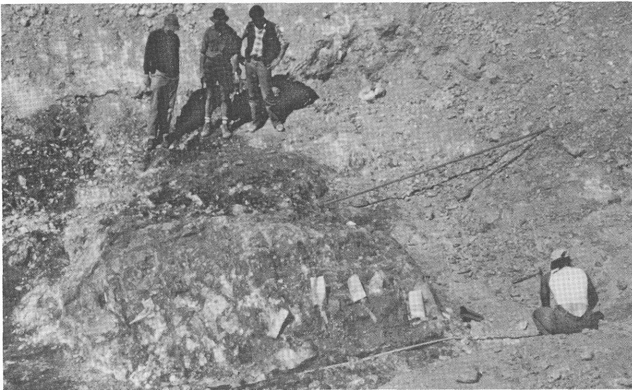
Plate 28. Massive sulphides of the Coronation zone exposed in trench on the Lara property (NMA87-28-01: 5414699N; 433574E). Photograph courtesy of H.P. Wilton. Results of the sampling taking place in the photograph are compiled in Appendix 2.
