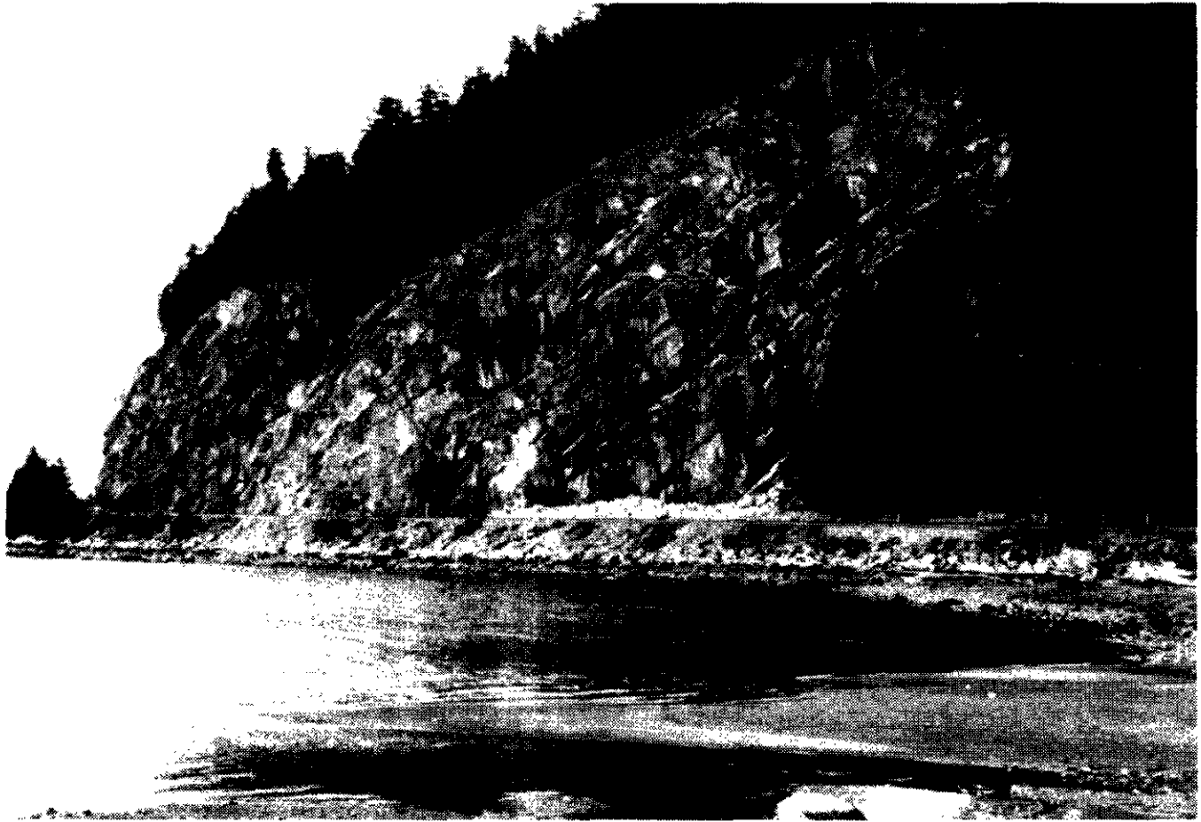
Plate 4-3-4. Sheet joints in quartz diorite bluffs at Porteau Cove along Highway 99, the site of a number of rockfall disasters. An ambitious slope-stabilization program was conducted at this site in 1991 by the Ministry of Transportation and Highways.
