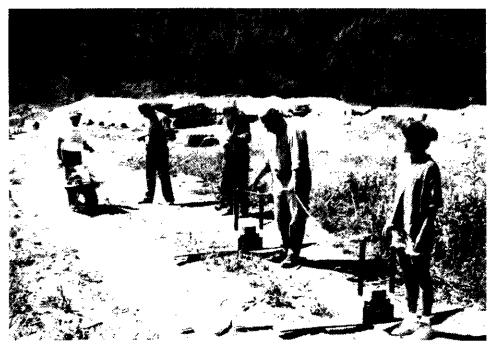
Plate 4-8-5. Equipment used for ground-penetrating radar surveys. Transmitting and receiving antennas, in the foreground, are connected by fibre-optic cables to the data collection and processing equipment in the background.
