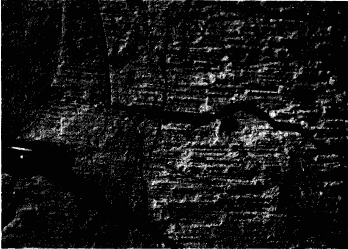
Photo 9. Joint surface in Tertiary rhyolite flow showing well developed striae generated by differential movement of lava blocks during flowage.
