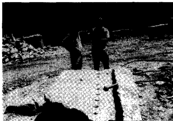
Photo 8. Cayoosh Creek quarry site - splitting the stone into masonry blocks
