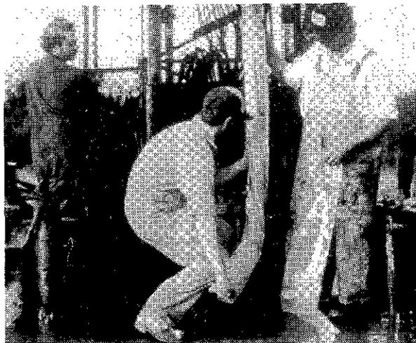
Photo 4-12. With the rotasonic drill, the core barrel is pulled to the surface and cores are retrieved in plastic sleeves in segments 1.5 metres long (GSC-1993-277-C).
