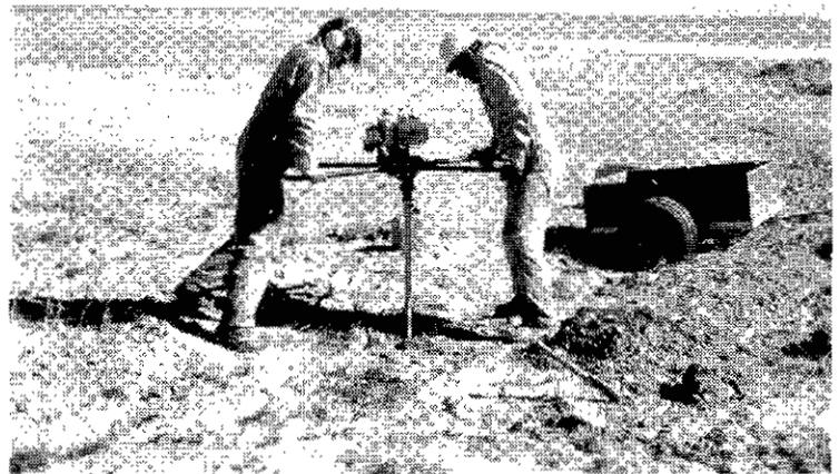
Photo 4-7. Stihl drill used by GSC in the high Arctic for permafrost sampling (GSC 202921-H).
