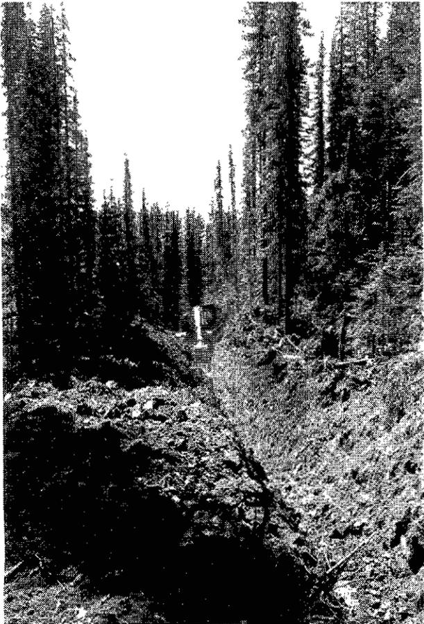
Photo 4-3. Two-metre deep trench dug down to bedrock. Note the excavator in the background.
