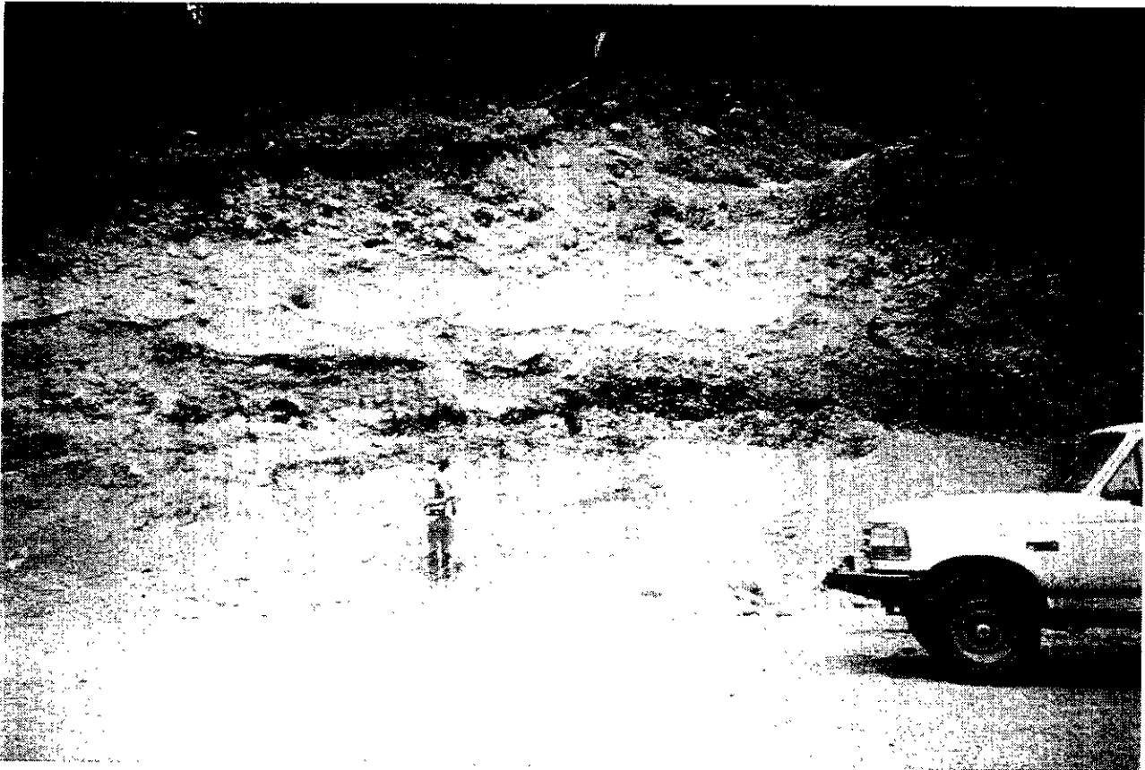
Photo 3. Borrow pit with greater than 30% fines.
