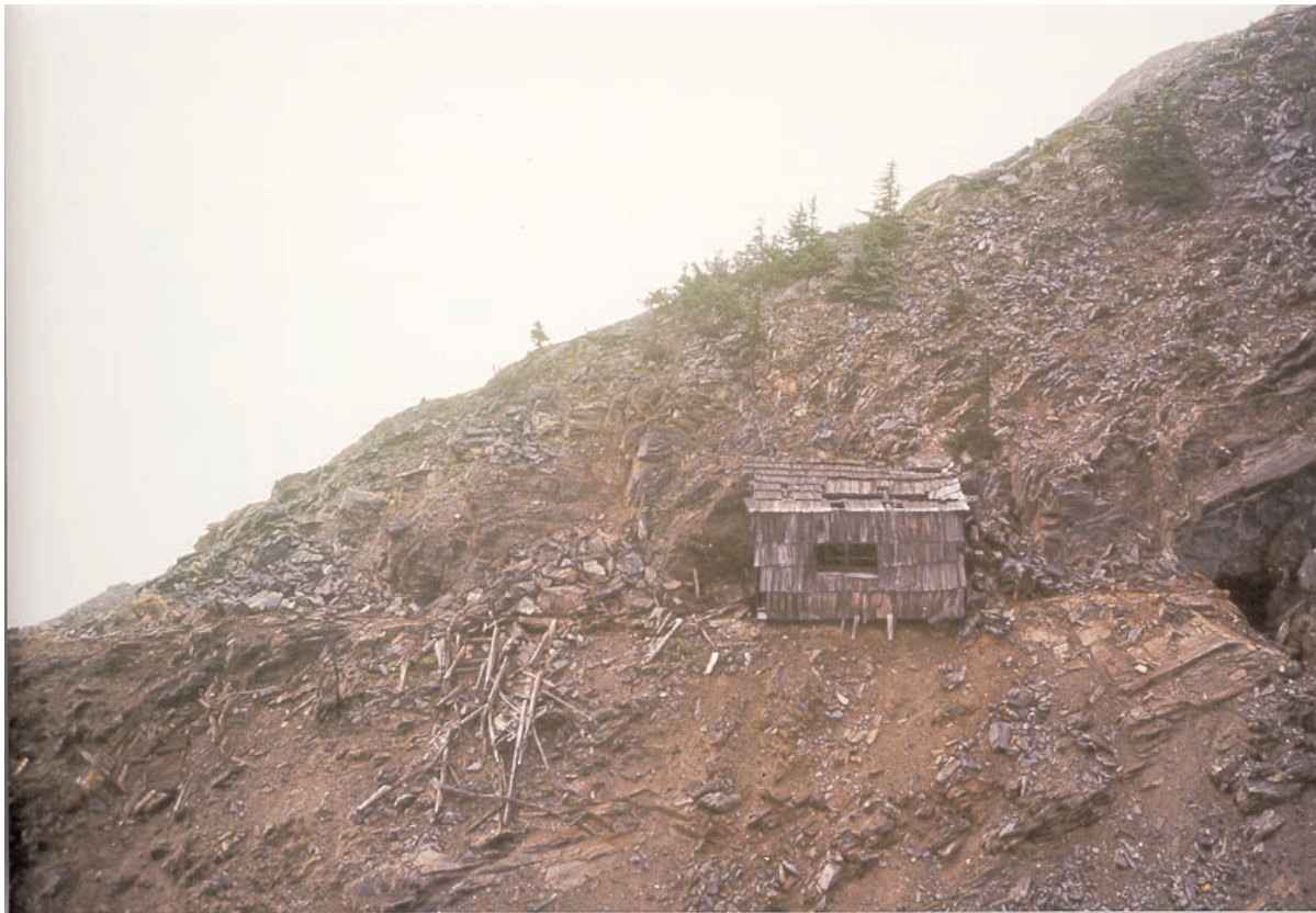
Photo 7. Main portal area, Mammoth mine, Mount Goldsmith.
