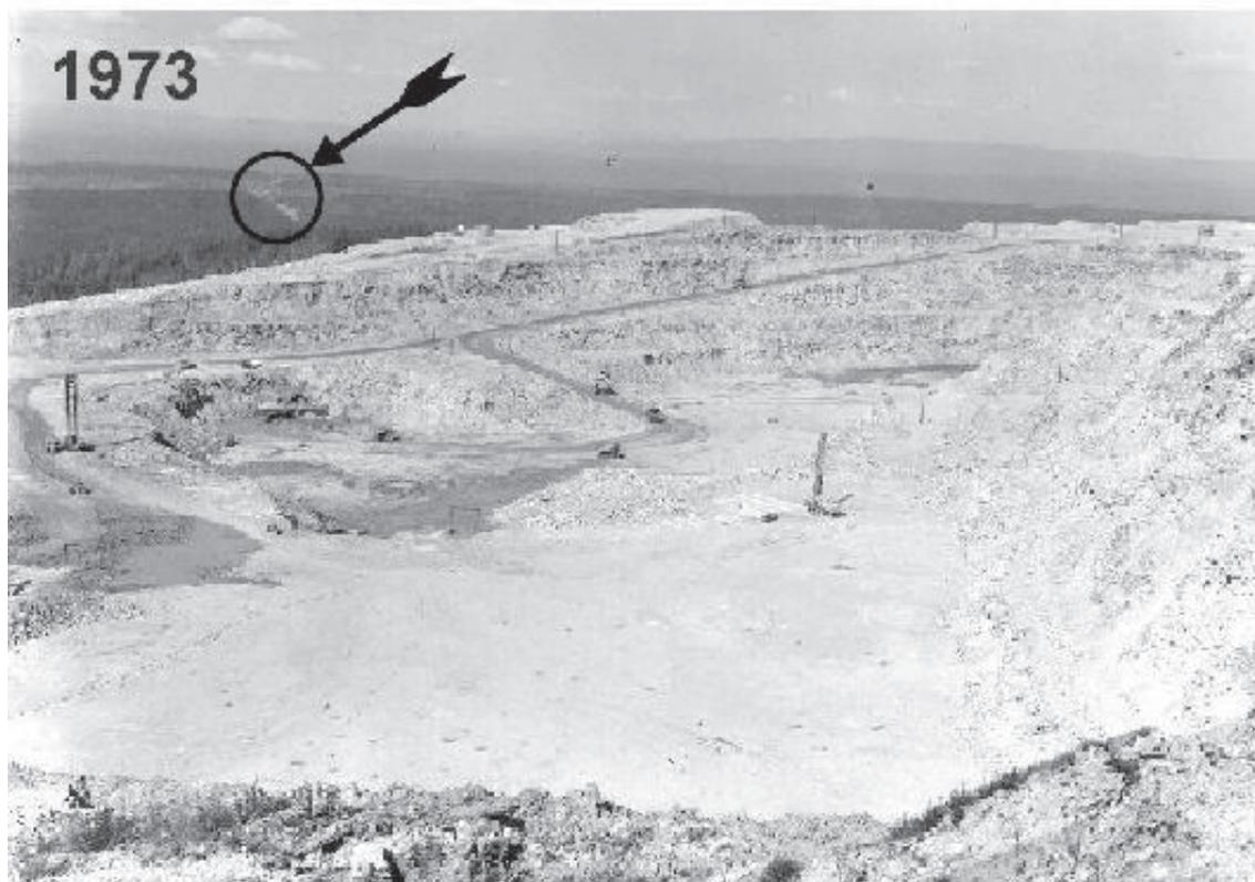
Photo 1. View of the Gibraltar East pit, looking west just prior to mine closure on the 2640 ft bench level in 1998 (top photo) compared to mining a year after start-up on the 3365 ft bench level in 1973 (bottom photo, Plate IV of Sutherland Brown, 1974). Circled area in background gives an idea of relative scale and position of the individual photos. Position of the pit in 1973 relative to that of the current pit outline is illustrated in Figure 3.
