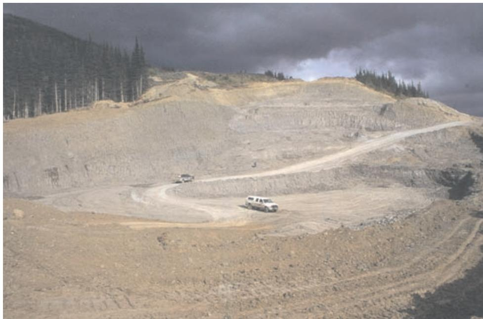
Photo 2. West Borrow Pit where till was excavated for use in tailings dam construction. This Pit was one of the 12 exposures studied on the Huckleberry Mine property. Note the trucks in foreground for scale.
