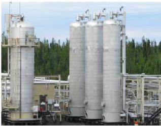
Figure 6. The Debolt water treatment facility taps the Mississippian Debolt Formation as a water source to ultimately support hydraulic fracturing operations. The Debolt is a deep, sub-surface, non-potable aquifer containing saline, sour water. This water source required many innovations including the investigation of several sweetening methods needed to remove the hydrogen sulphide and make the water usable.
