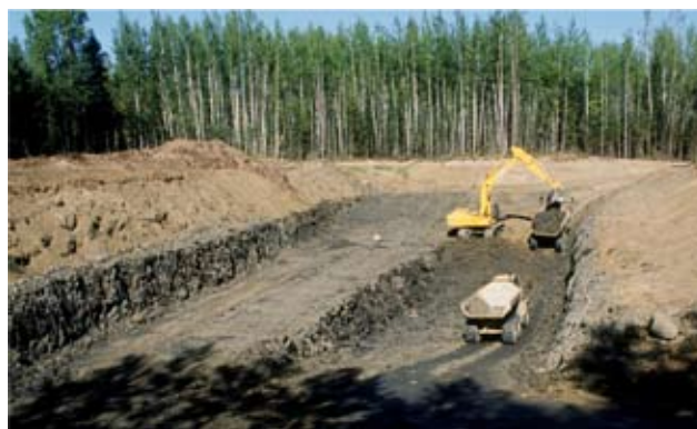
Figure 4. Excavation of till from a borrow pit for construction of a well site access road. Photo R. Smith.
