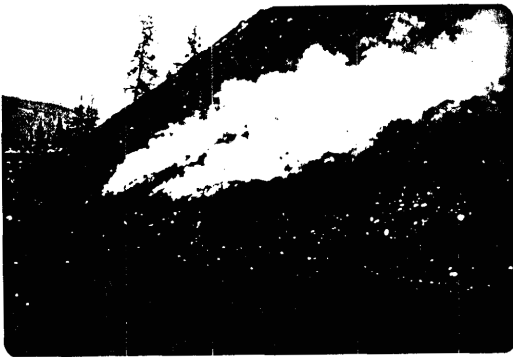
3. Fire in uncrushed low grade pile August 27/77
