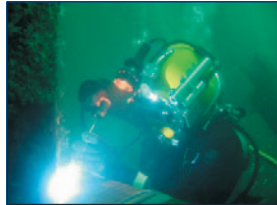
Coded wetwelder/diver repairing marine structure
