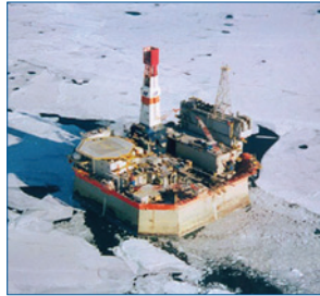
Refurbishment and deepening of the Sandwell-designed Molikpaq arctic structure
