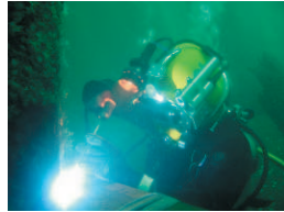
Coded wetwelder/ diver repairing marine structure
