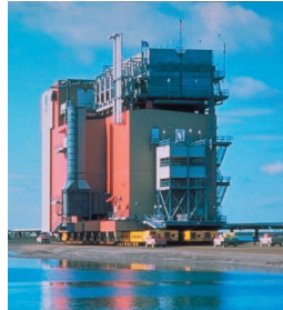
Sealift Module from VECO's Anchorage Shop
