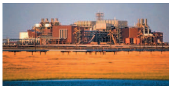
BP Milne Point Production Facility in Alaska
