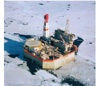
Refurbishment and deepening of the Sandwell-designed Molikpaq arctic structure
