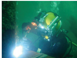
Coded wetwelder/diver repairing marine structure
