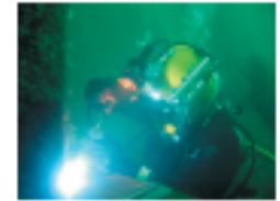
Coded wetwelder/ diver repairing marine structure
