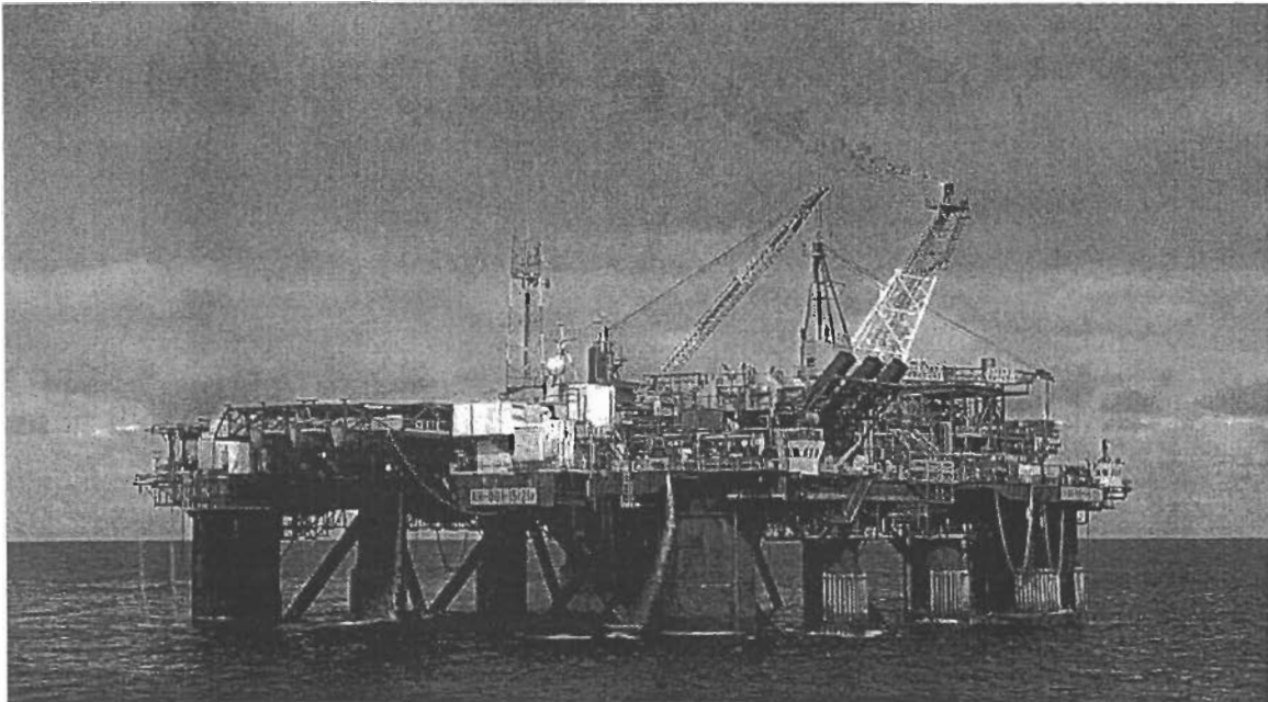
North Sea Platform at Work
