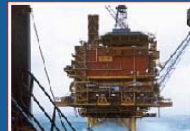
Steel Jacket Platform
