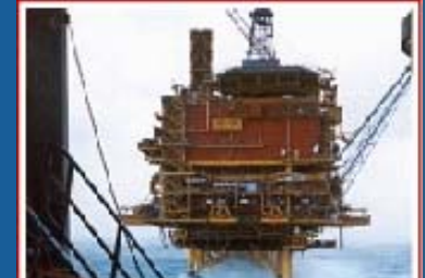
Steel Jacket Platform
