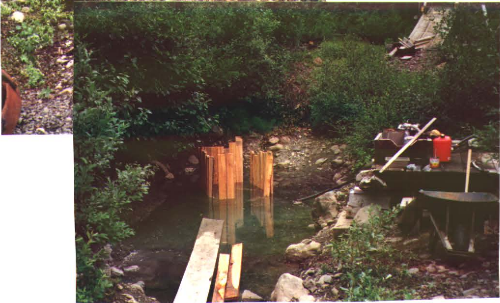
MIDDLE & BOTTOM PICTURE Example's of the high water problem.
