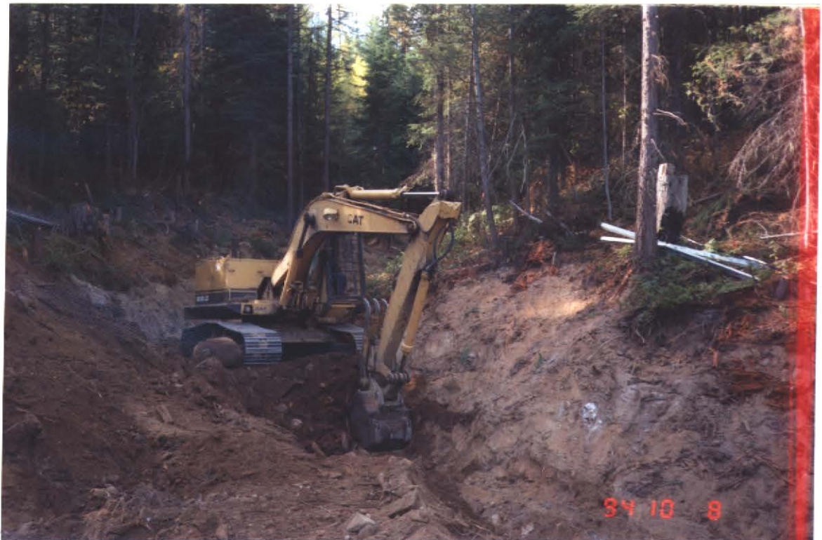
Photo 17- the start of the excavation at Site " D"
