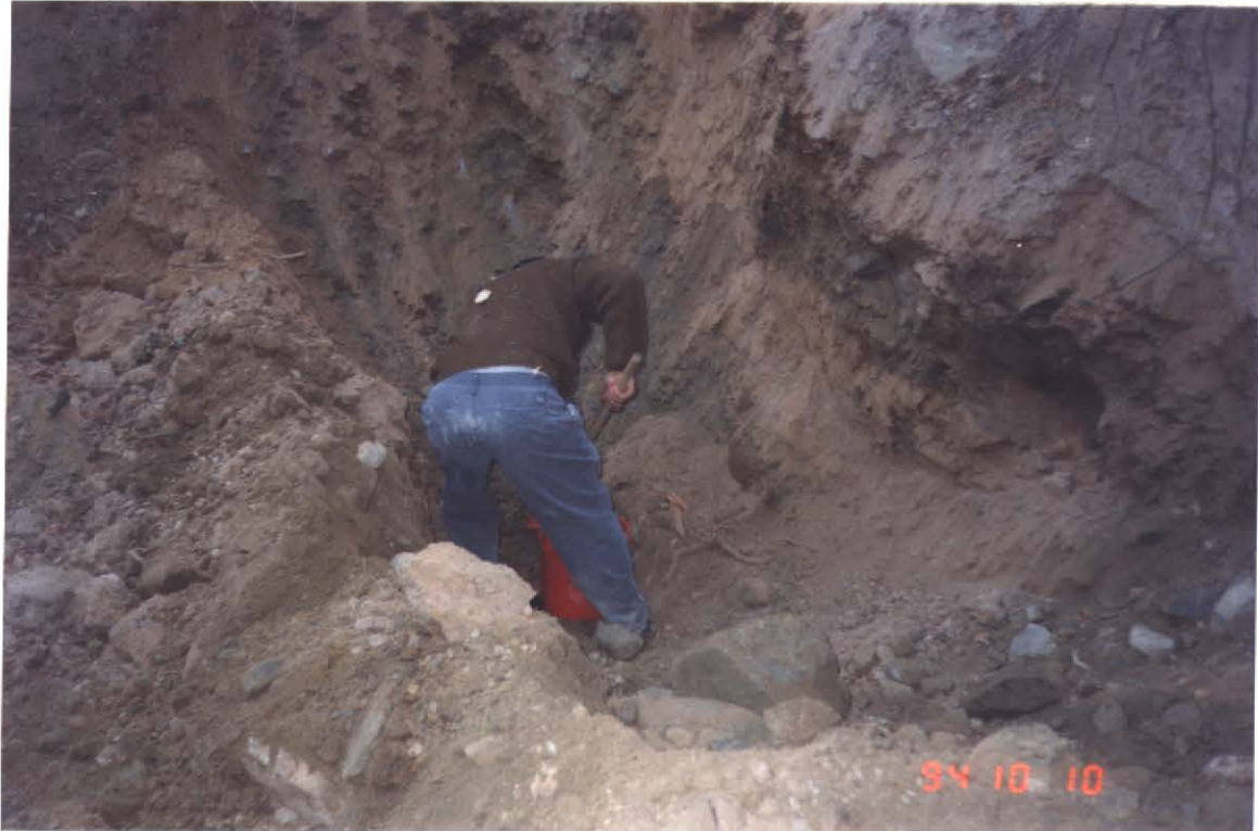
Photo 22- Hardpan or densely packed and cemented gravels, could have been early glacial deposits, These hardpans were almost impossible to work loose without heavy machinery
