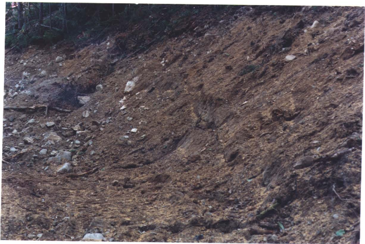
Photo 29 - Slopes Backbladed with the Cat 225
