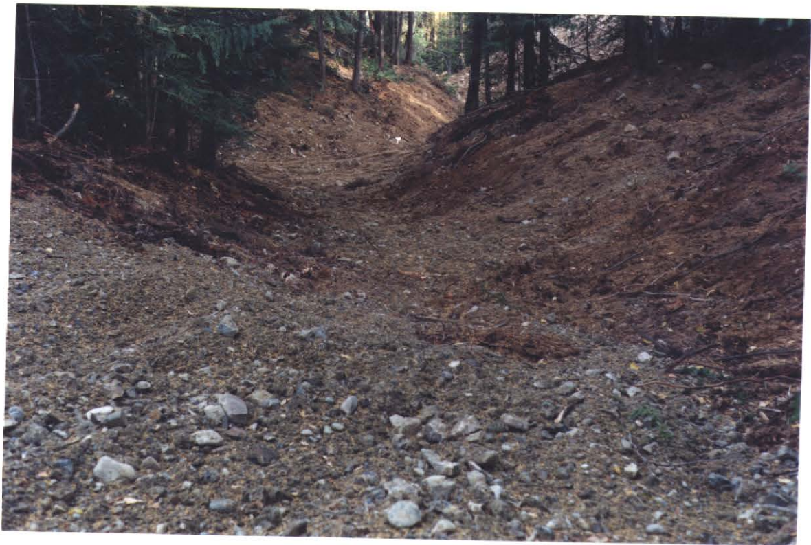
Photo 28 - Looking down the primary gullie, the Excavator contoured the slopes of the holes as close to 2:1 as possible. This photo is looking down on site "E"
