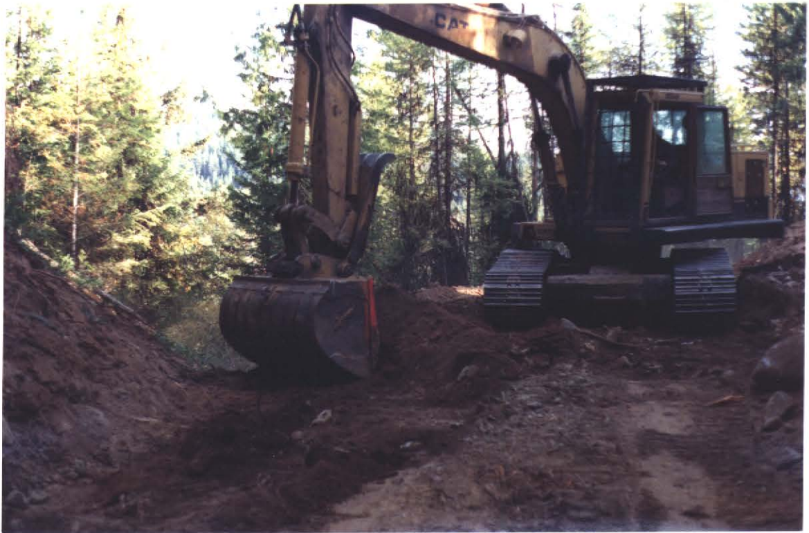
Photo 14- The cat excavating at Site "B"
