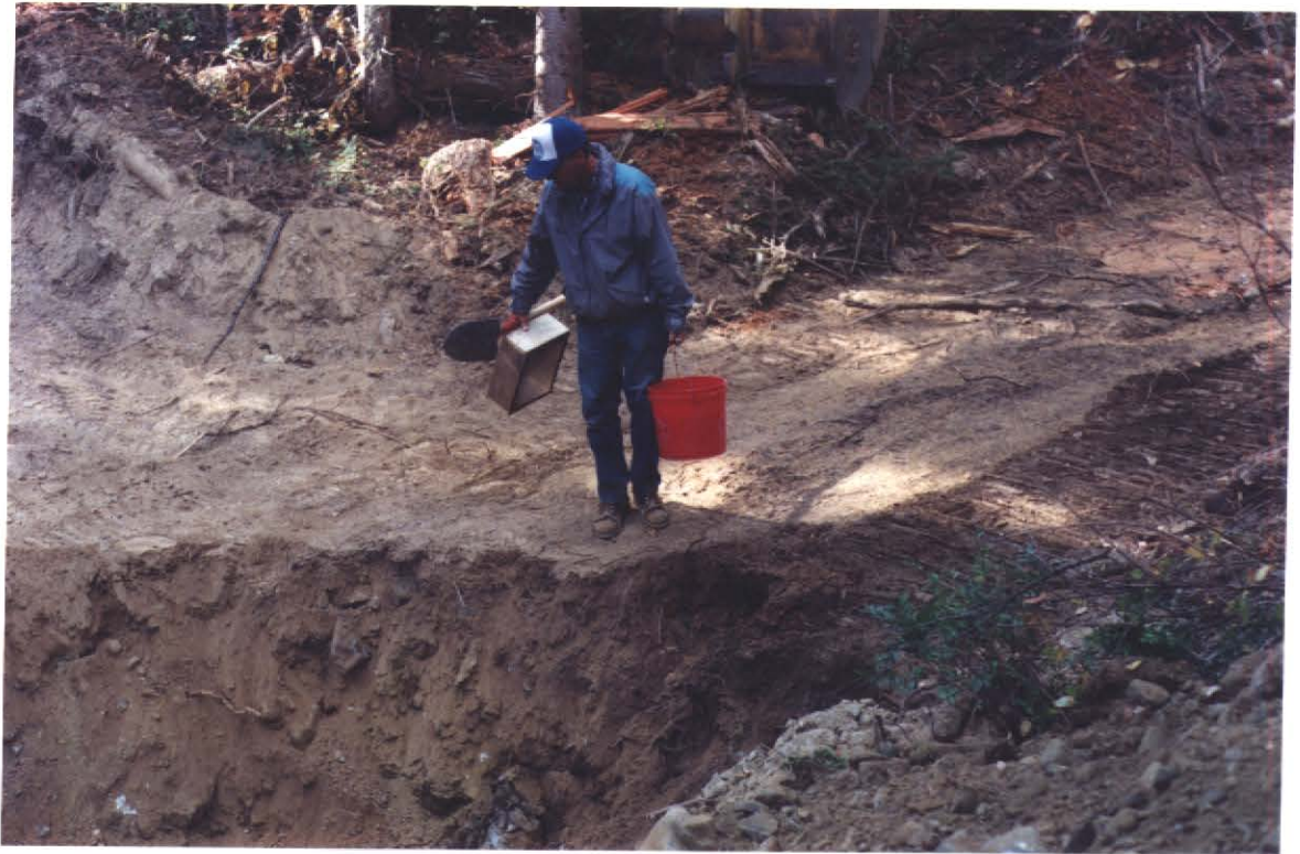
Photo 24- Material was bucketed out of the excavations or in the deepest depths was sampled with the Cat bucket
