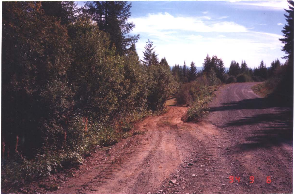
Photo10- The old existing logging road was graded for about 500 meters from its start at the old Phoenix Road
