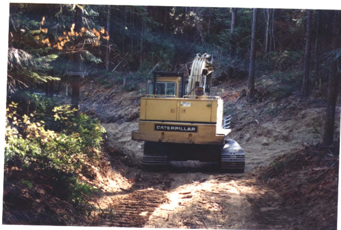
Photo 13- The Caterpillar 225 ready on 94-10-07 to excavate the sample holes.
