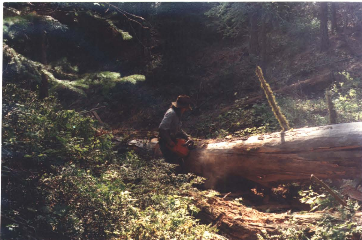
Photo 5- A contract faller was hired to fell about 12 danger trees before heavy equipment could be brought in
