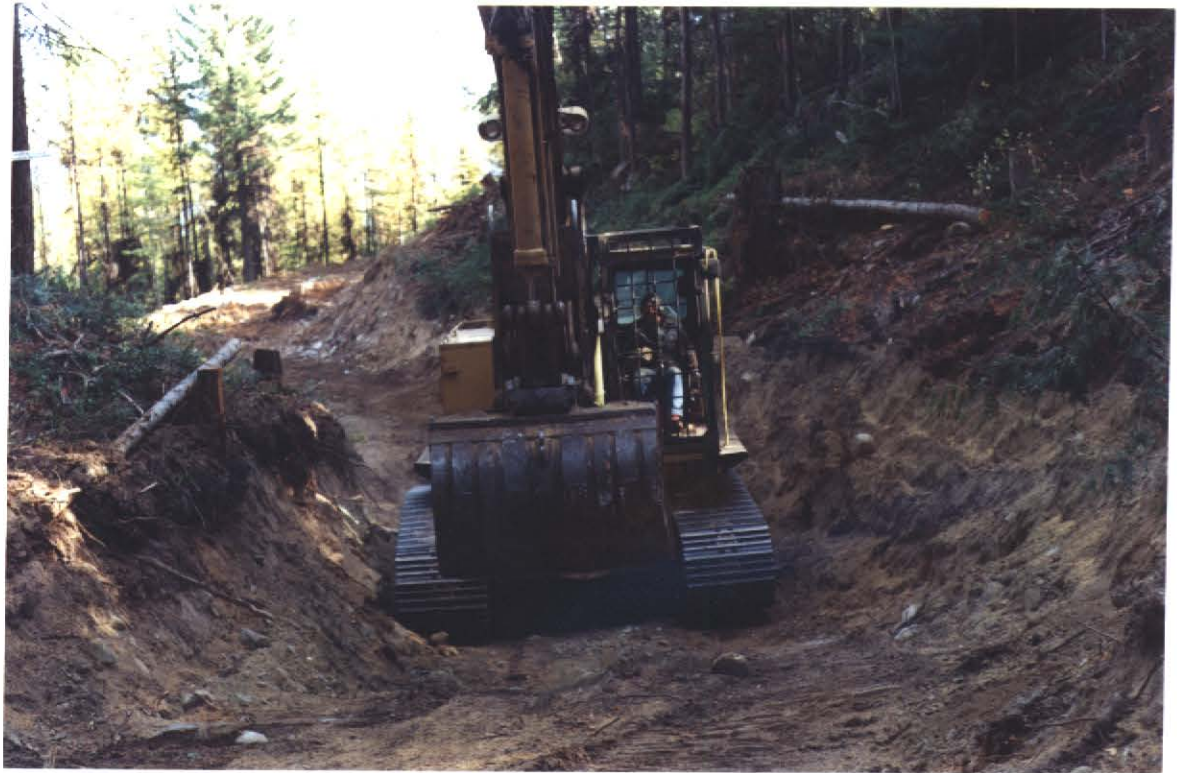
Photo 15 - The cat on 94-08-08 starting the excavation of Site "C"
