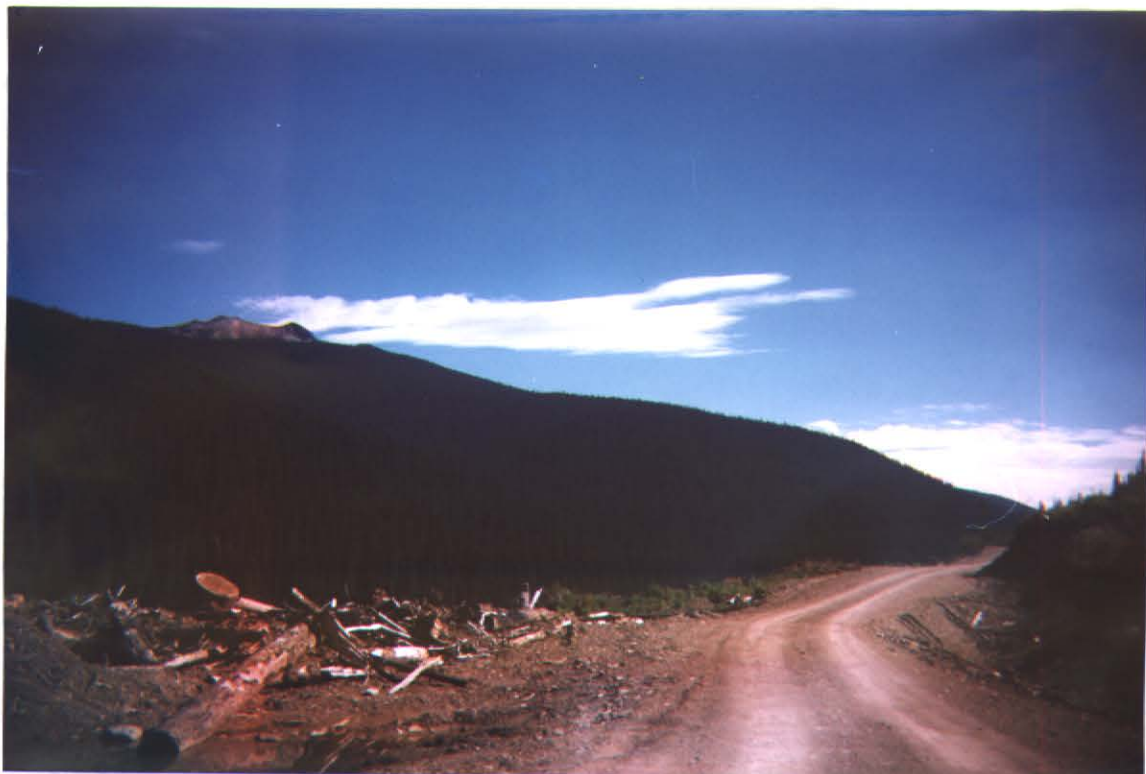
APPROACHING CUNNINGHAM CREEK (UPPER) ALONG 3100 'N' ROAD.
