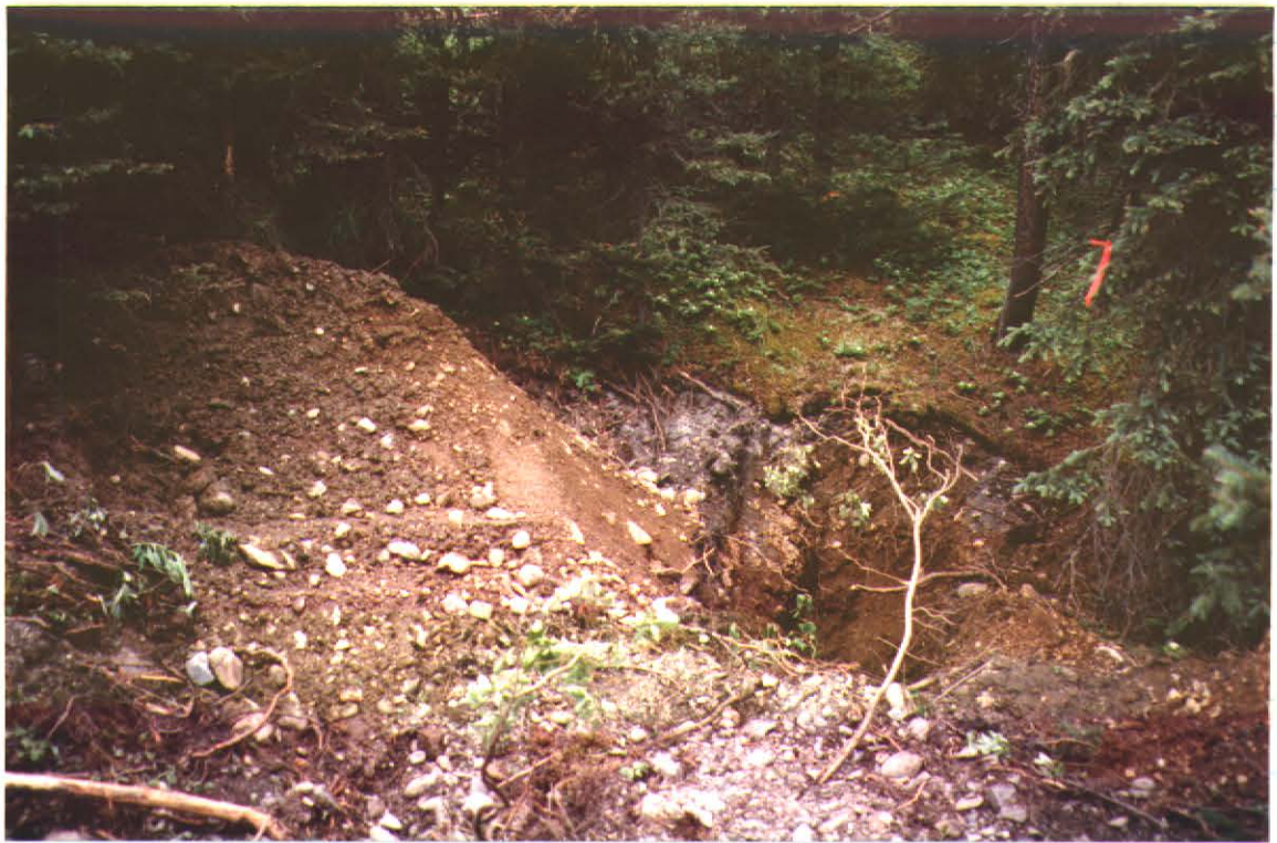
Typical test hole approx. 3m deep
