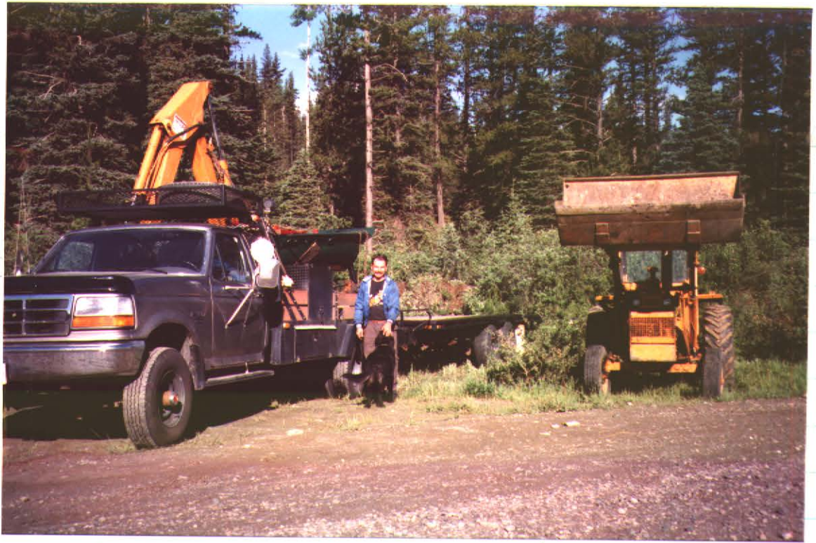
Unloading Equipment At Canadian Creek (2 trip)
