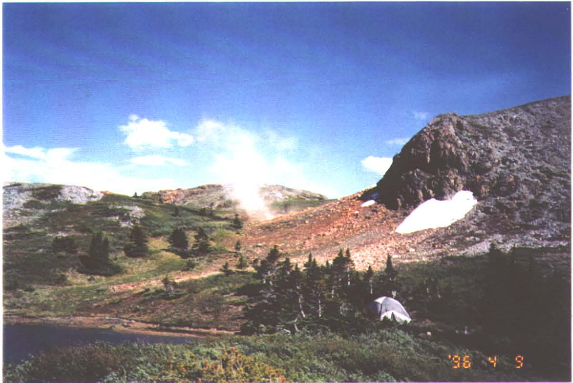
BLASTING TRENCH NUMBER 1 IN BLUE BIRD FAULT.
