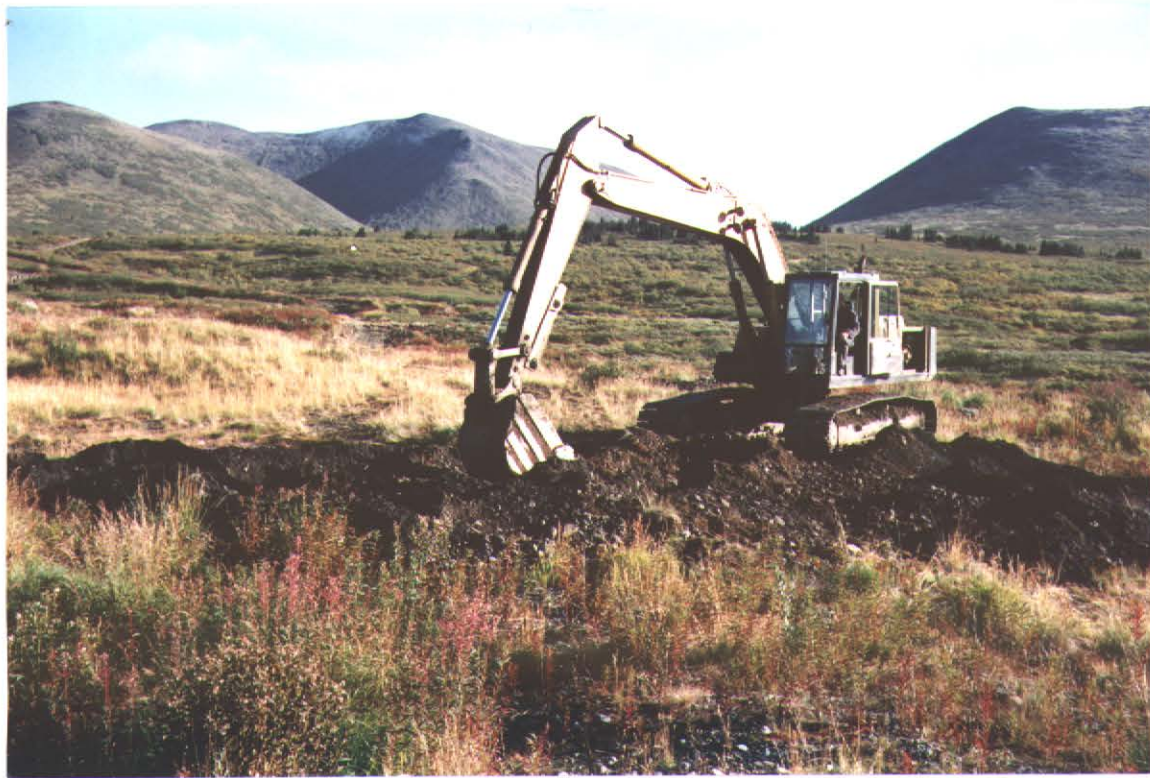
EXCAVATOR @ WORK. DIGGING TEST HOLES APPROX. 20' DEEP. SITE #5
