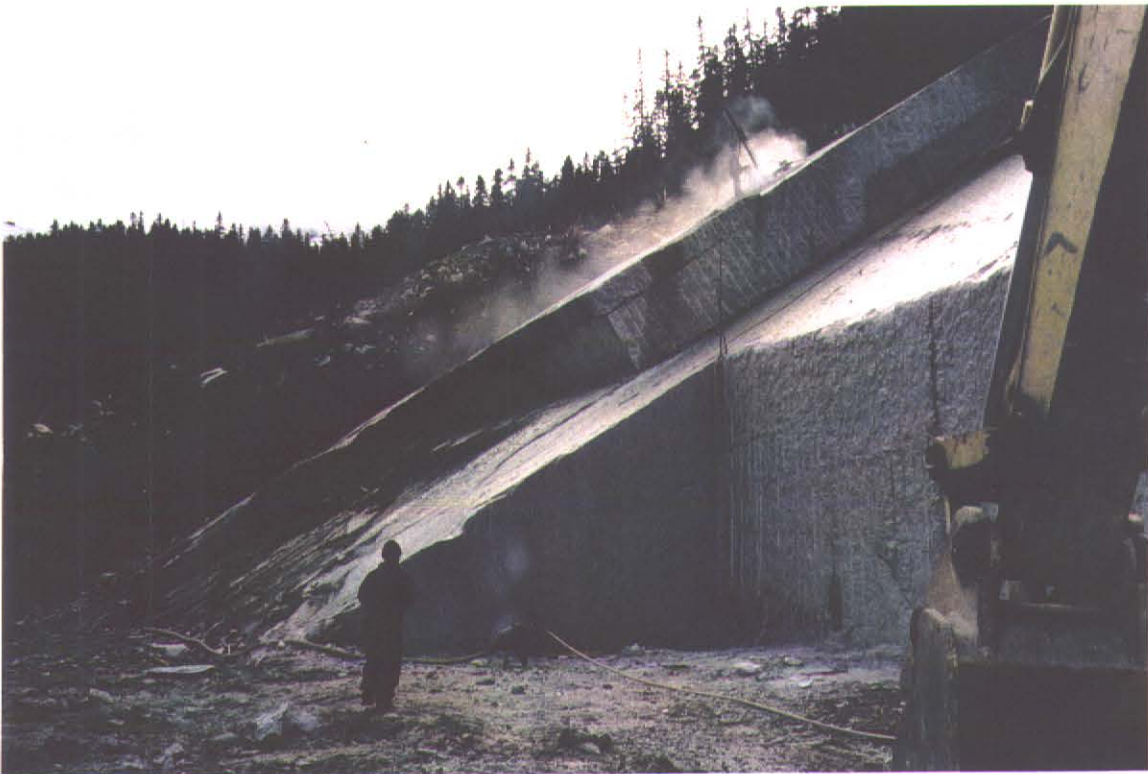
Photo 4.4 - East Anderson River Quarry
