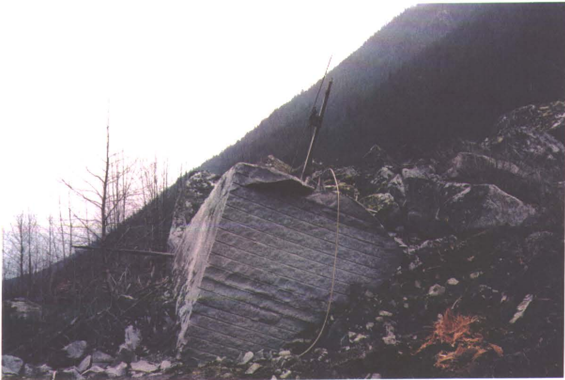
Photo 3.4.c - Circa 30 tonne boulder being drilled.
