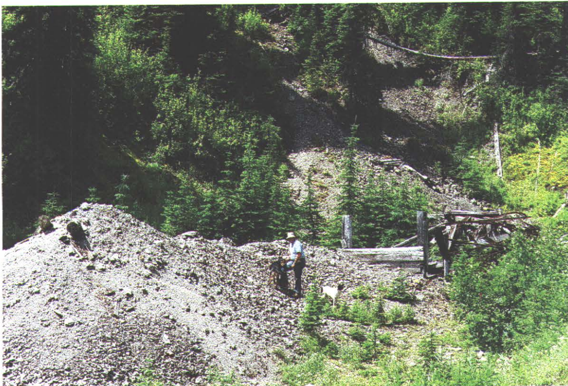
Fig. 2. Shannon (MINFILE 082KSW060), with ore stockpile in foreground, collapsed portal in background.
