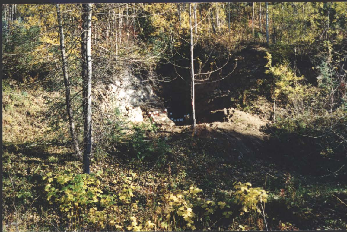
Photo 2. Jack Rabbit fault looking south east showing collapsed adit circa 1928.
