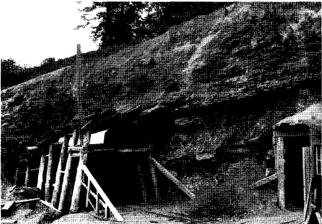
B. Outcrop of fireclay-seam and portals of underground workings of Richmix Clay Company, near Kilgard.
