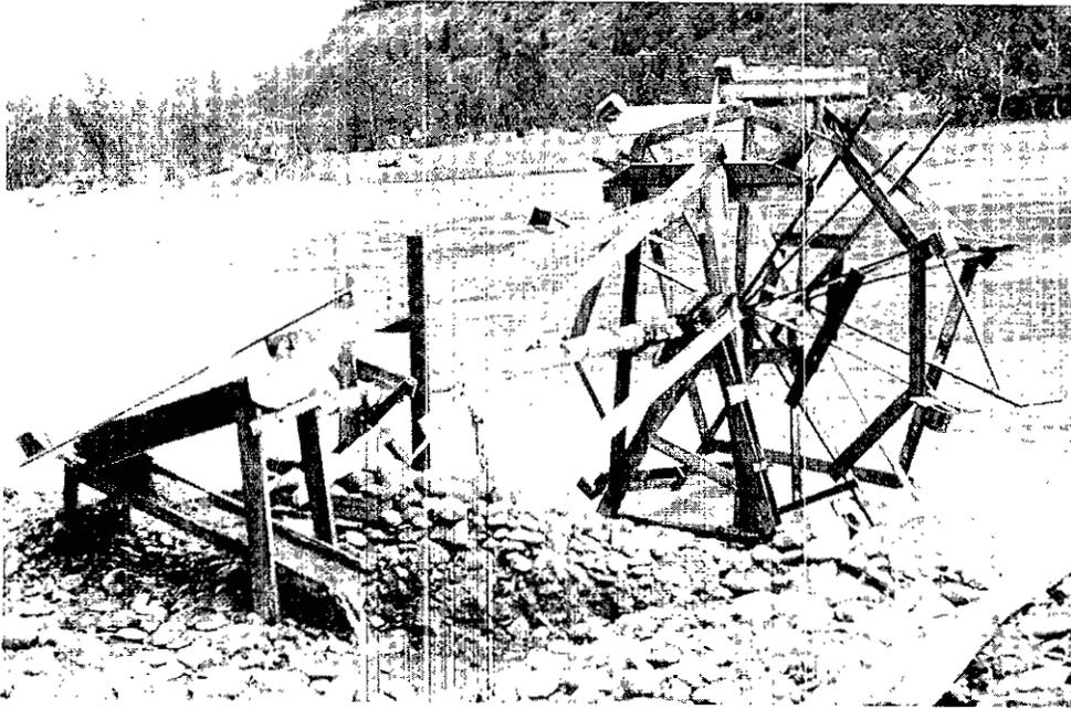
A. A simple and easily constructed current wheel delivering water to a short sluice on the Fraser River below Quesnel.
