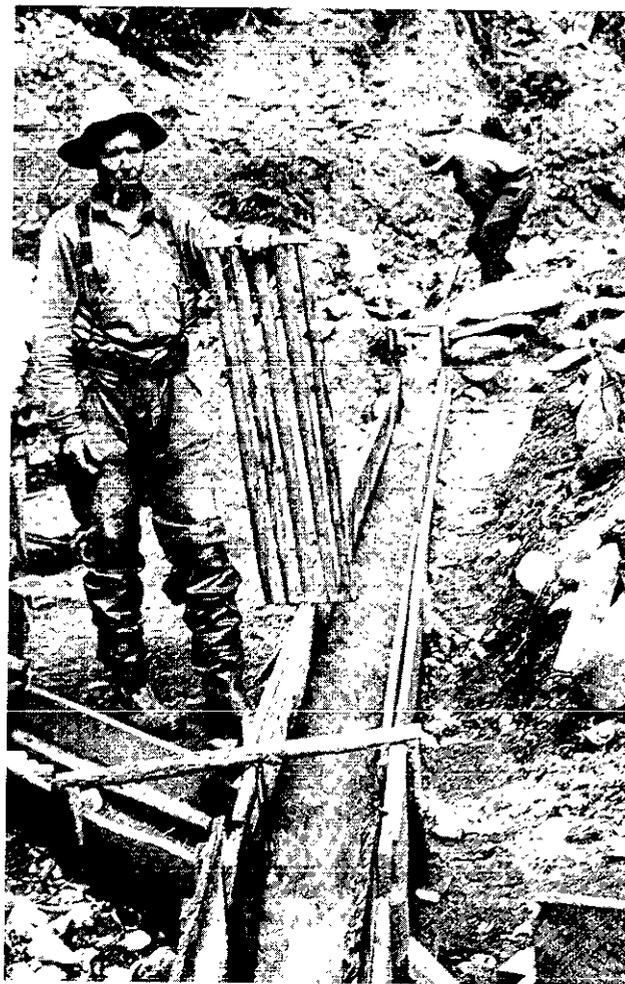
B. Sluice-box set up for shovelling-in. A section of pole-riffles is shown.
