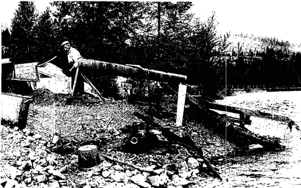
B. A portable placer-pump delivers water to a metal trough which discharges the gravel onto a shed grizzly. The undersize is washed in the sluice-box at the extreme right. The gravel is brought by truck from a low bench beside the Tulameen River.
