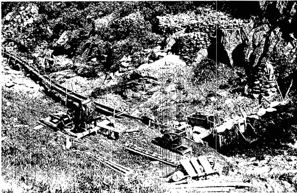
B. Shovelling-in operation on Alice Shea Creek. The entire creek flows through the sluice-boxes. Notice the rock-piles in the background and the hoist and portable pump in the foreground.
