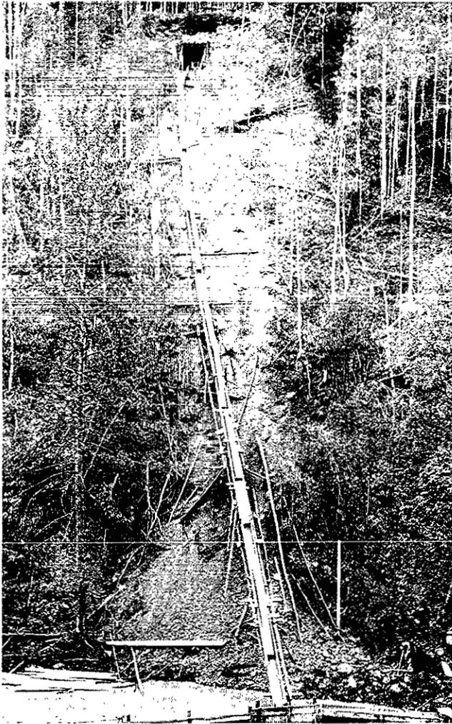
A. A bench mine with a gravel-slide from the portal of the drift to sluice-boxes set up in the creek.
