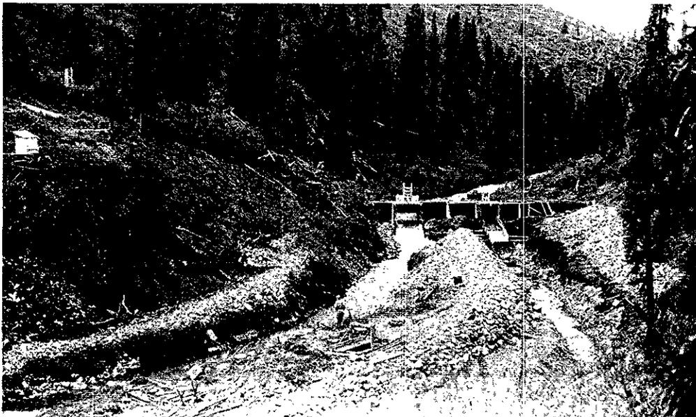
B. Boom dam and ground-slucice cuts on Wheaton (Boulder) Creek. The cuts are worked alternately. Large boulders are thrown from the cuts and the smaller gravel is washed through.
