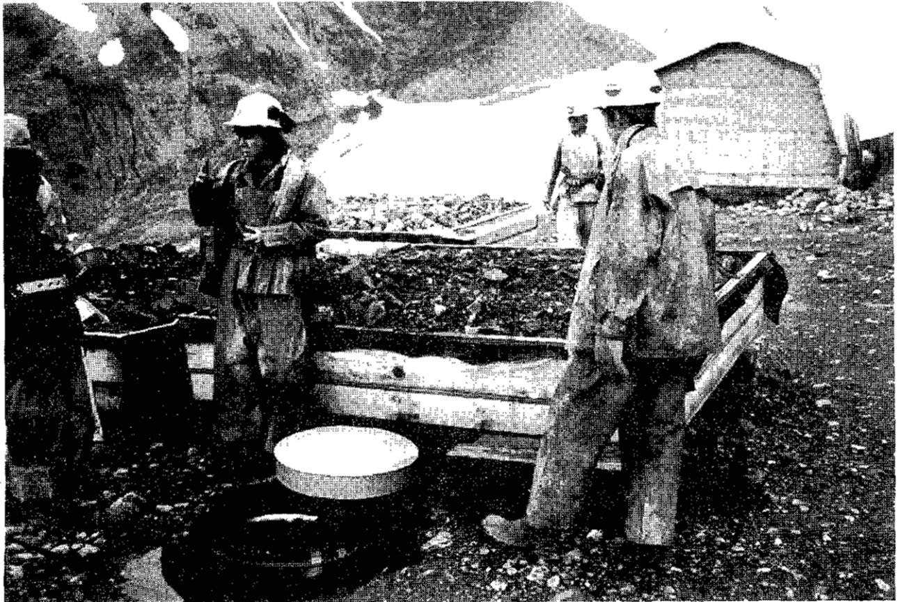
Plate A-1. Geddes Resources Ltd. continued to work on developing the huge Windy Craggy copper deposit. The company completed numerous studies to assess the impact of a mine in this remote location, including field tests on the potential for developing acid drainage shown in the picture above.
