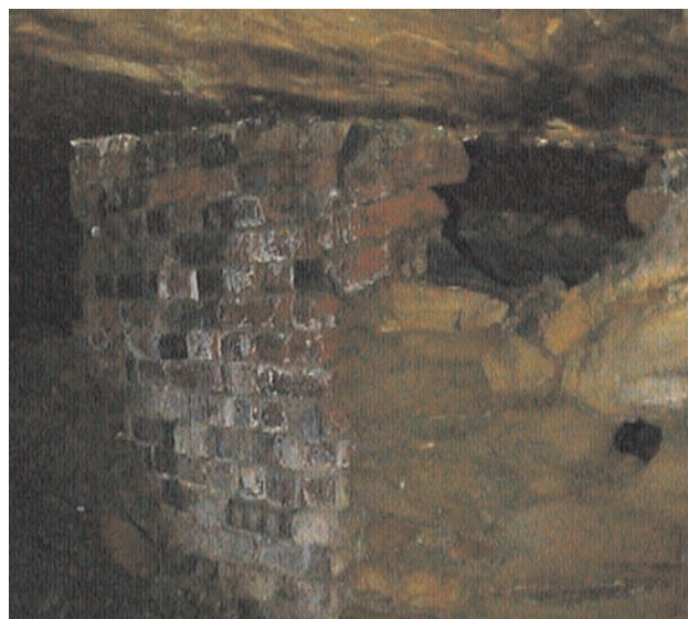
Photo 2. Original firewall of brick and stone, on north side of underground ventilation furnace, inbye Portal 5. Sandstone roof above furnace has been baked and reddened, and shows minor flaking.
