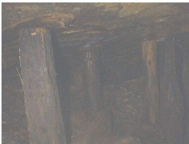
Photo 1. View southward into workings inbye Portal 4. Timber posts are 20 to 30 cm in diameter, and have single cap-pieces to spread load against carbonaceous mudstone roof of coal bed.
