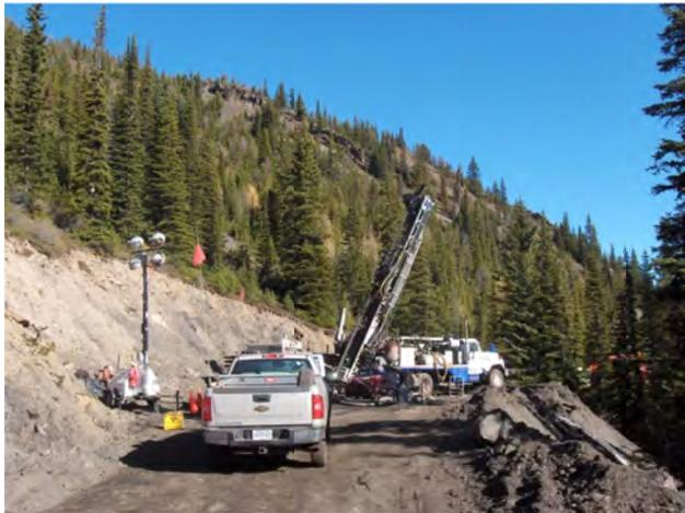
Figure 19. Rotary drilling on Teck Coal Limited's Burnt Ridge North property.
