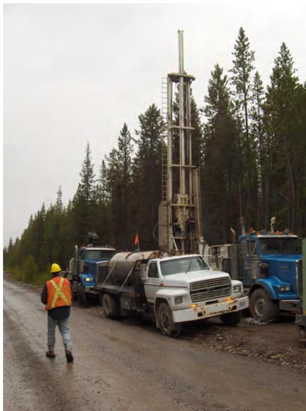
Figure 17. Rotary drilling at the side of the Elk Valley Forest Service Road north of Elkford on Centremount Coal Ltd's Bingay Creek coal property.
