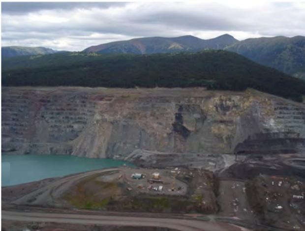
Figure 2. Kemess South mine showing failures on the north wall that result from graphite-bearing Asitka Group sedimentary rocks. A basement “high” of Takla rocks separates tailings in the West Pit from active mining in the East Pit.
