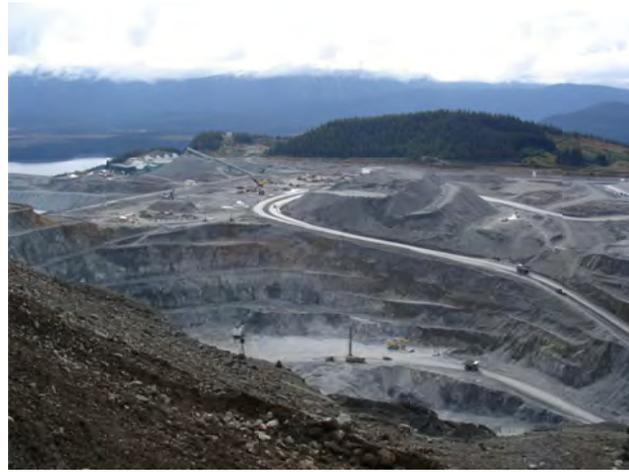
Figure 6. Huckleberry copper mine; mining in the MZX pit in September 2010, low grade stockpile and mill in the background.
