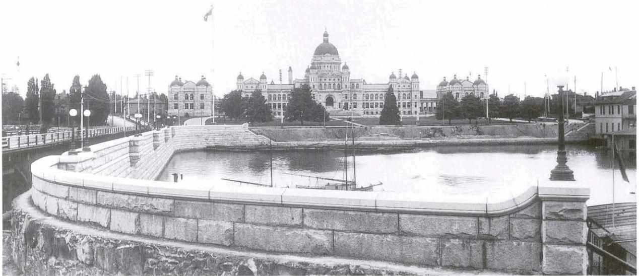
*Photo of the Inner Harbour, Victoria, B.C., 1906 Shows the Legislature building with the newly completed seawall in front of the James Bay Bridge. The seawall (page 13) is part of a cofferdam which cut off the western reach of the harbour. This was done so that the Empress Hotel could be constructed on what was then the James Bay mud flats. Photo from B.C. Archives and Records Service, Catalogue No. 56023.*
