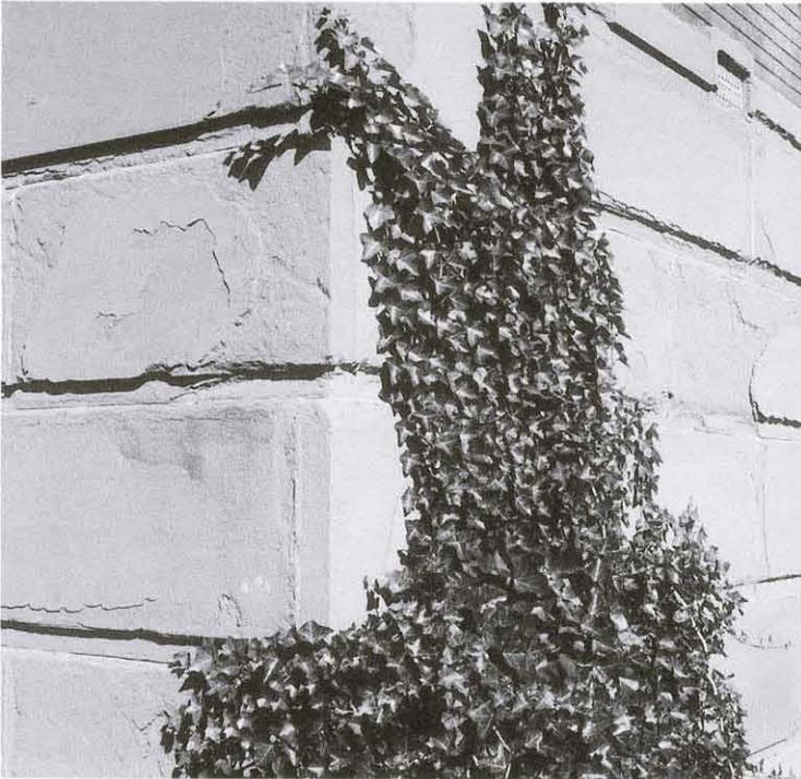
*Continuing decay of the Denman Island sandstone in these pillars on the Camosun College campus in the form of cracking and stripping is due to the effects of rain and frost on the vertically exposed bedding planes.*
