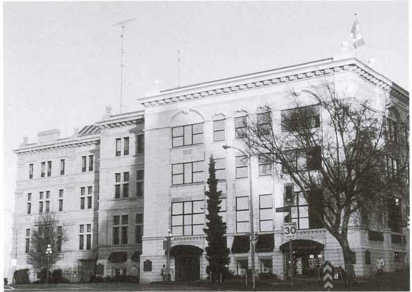
*“ ... Both rock-face and bushed work have weathered well, but certain blocks show evidence of disintegration. It is said that this defect is due to the use of material which had been soaked in salt water.... On some of the smoothed work there is a strong tendency to brownish staining.... Individual blocks are already showing disintegration; but it appears a more careful selection of the stone would have obviated this defect....” (Parks, 1917)*
