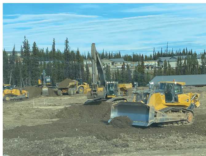
Fig. 4. Construction activities at the Blackwater Gold project site (Artemis Gold Inc.).
