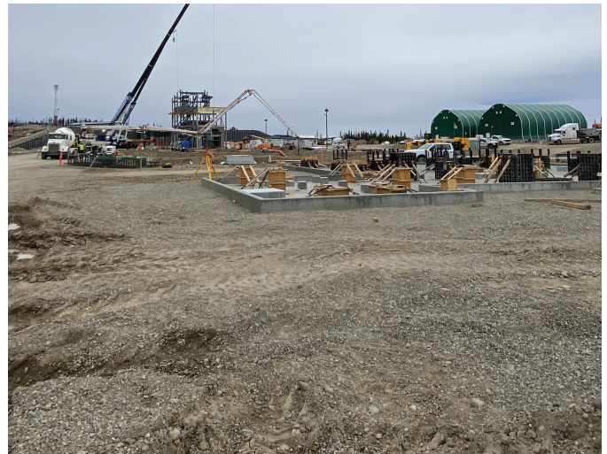
Fig. 5. Construction activities at the Blackwater Gold project site (Artemis Gold Inc.).
