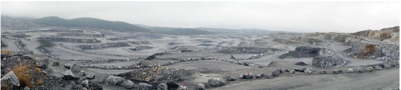
Fig. 4. Texada Quarry on Texada Island (Lafarge Canada Inc.).
