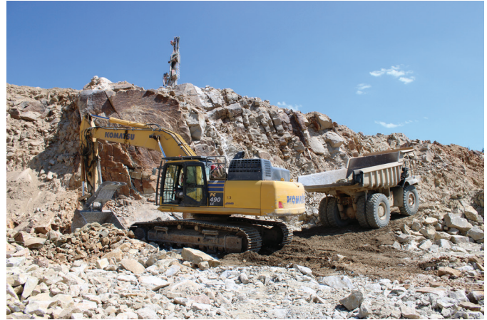
Fig. 2. Blast hole drill, excavator, and haul truck at Elk Gold mine (Gold Mountain Mining Corp.).
