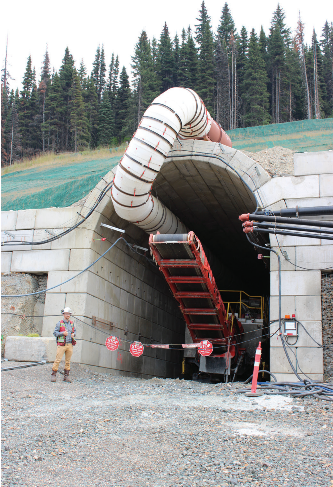
Fig. 3. Cow Mountain portal at Cariboo Gold project (Osisko Development Corp.).
