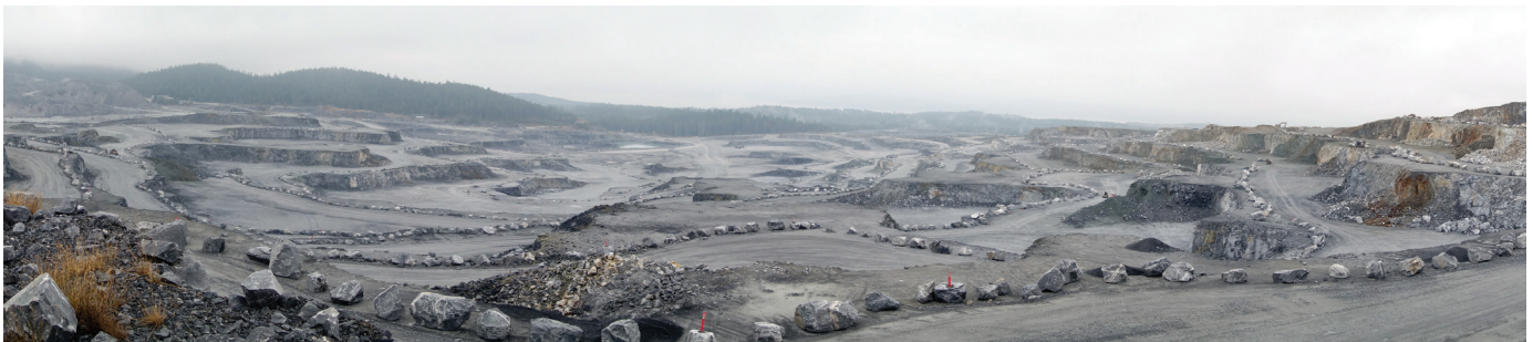
Fig. 2. Lafarge Canada's Texada Quarry limestone operation on Texada Island.
