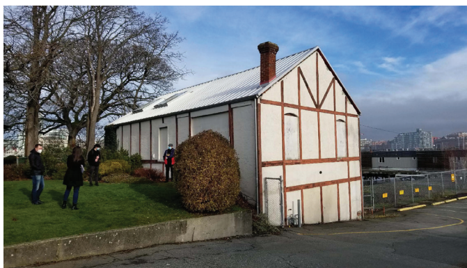
Fig. 1. Heritage 'Stores Building' (ca. 1912) at 254 Belleville Street, Victoria.
