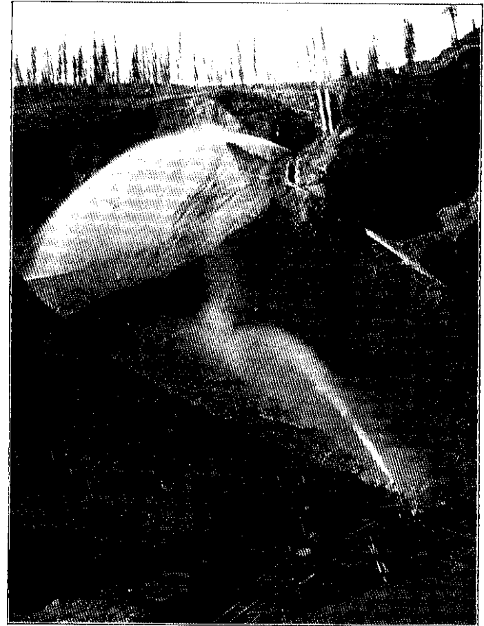
HYDRAULIC WASHING WITH MONITORS—CONSOLIDATED CARIBOO HYDRAULIC MINING CO.
