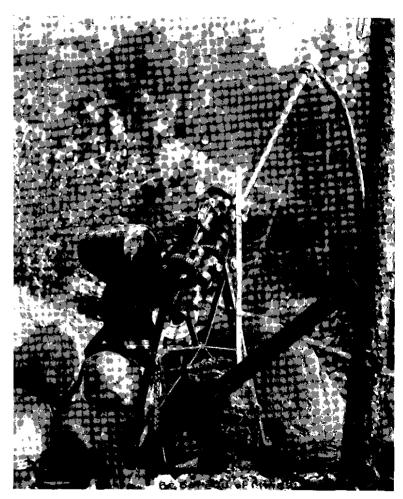
Union Mine, Grand Forks-Light Portable Diamond-drill for Surface Operations.
